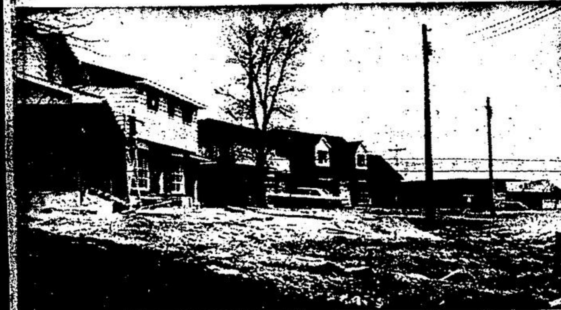
A NEW STREET IS BEING CREATED IN THE Lane orchard subdivision. This row of new homes by Dax Construction is part of the new development of Carole Street.
