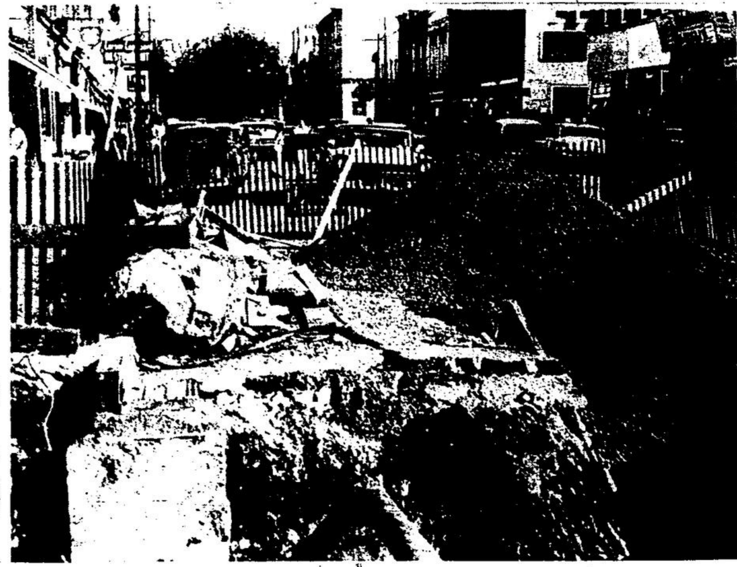
GEORGETOWN'S subterranean river which at one time provided the town's drinking water supply is the object of this attack from the surface on Main St. N. Inspection showed the river's man-made channel was slowly collapsing and instigated this operation which will replace the damaged tile. The inspection and repair work are first steps on Main Street reconstruction.
