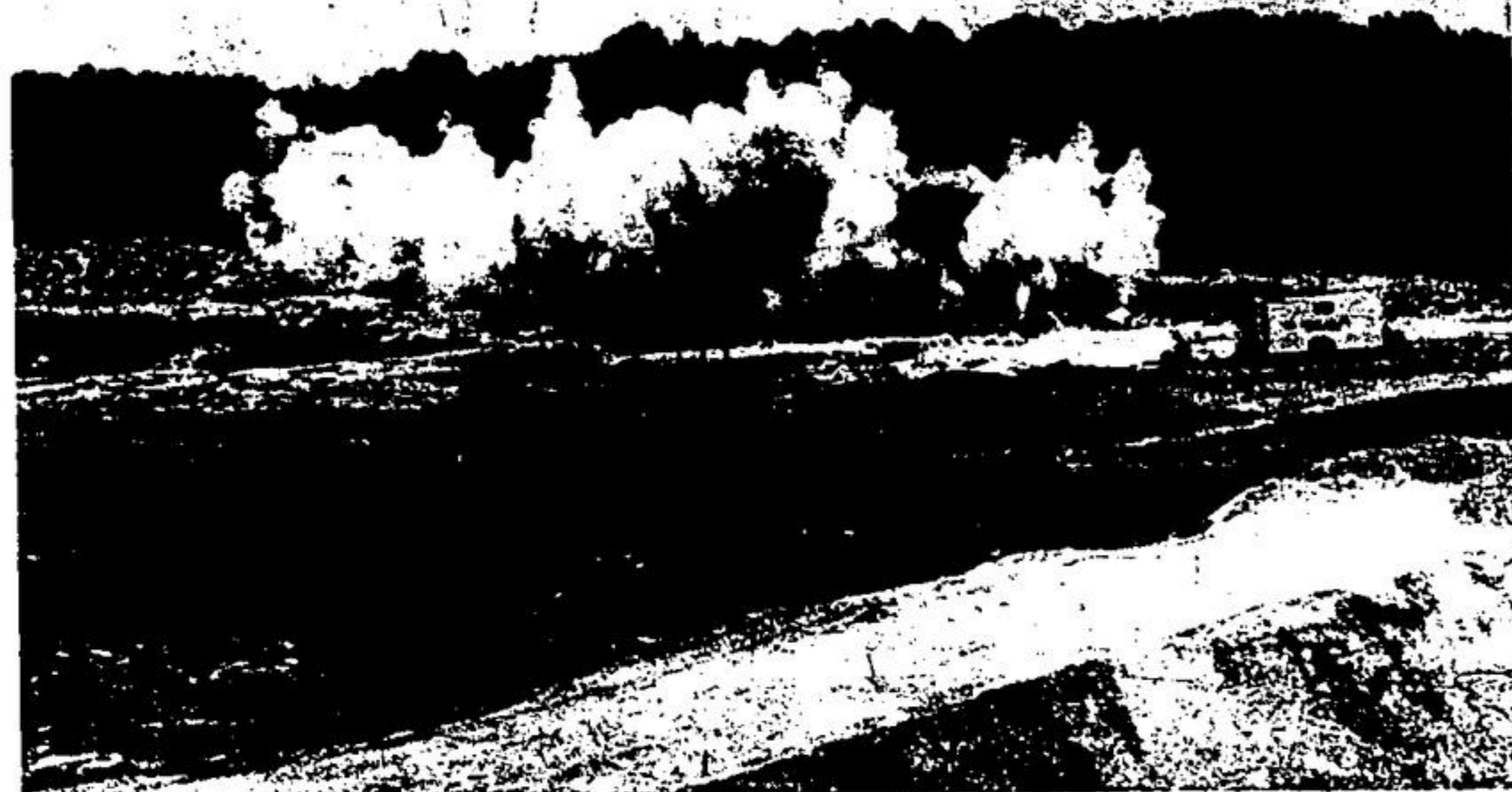
AFTER THE DRILL HOLES are loaded with dynamite the charge is detonated. Seven thousand tons of rock were blasted in this photo
