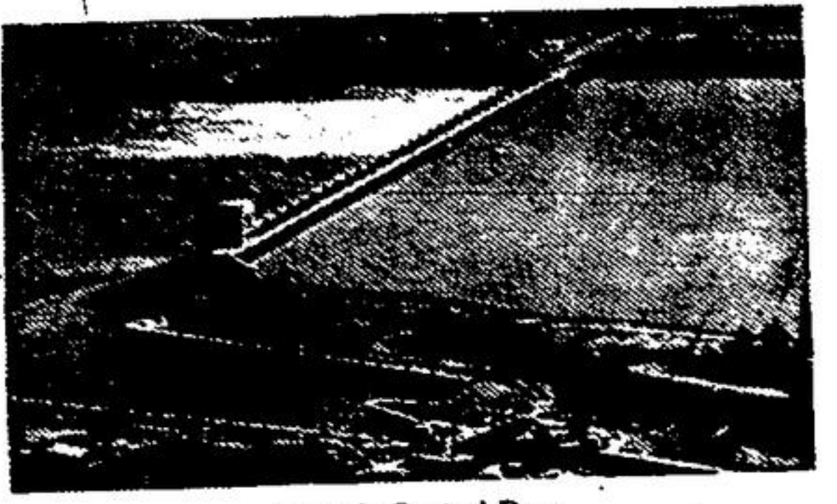
Iroquois Control Dam
