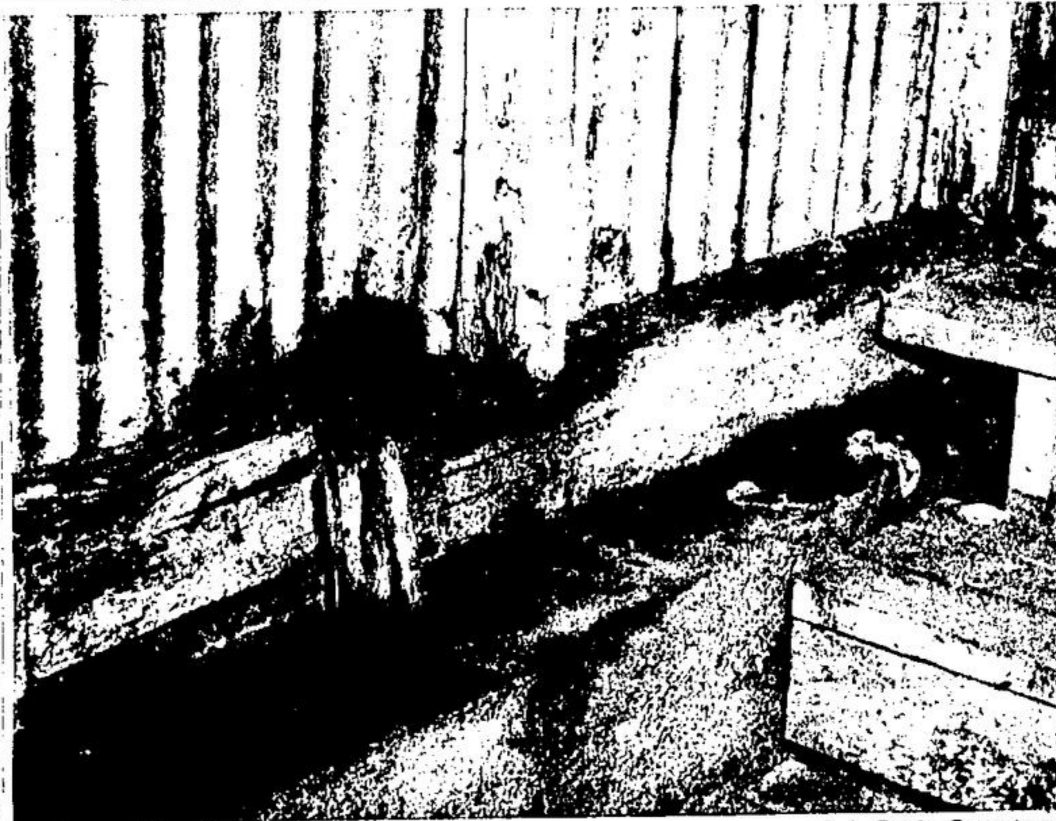
SERIOUS DETERIORATION of the footings in Georgetown Memorial Arena is shown in the photo above. The proposed renovations will eliminate this dangerous condition which is steadily growing worse.
