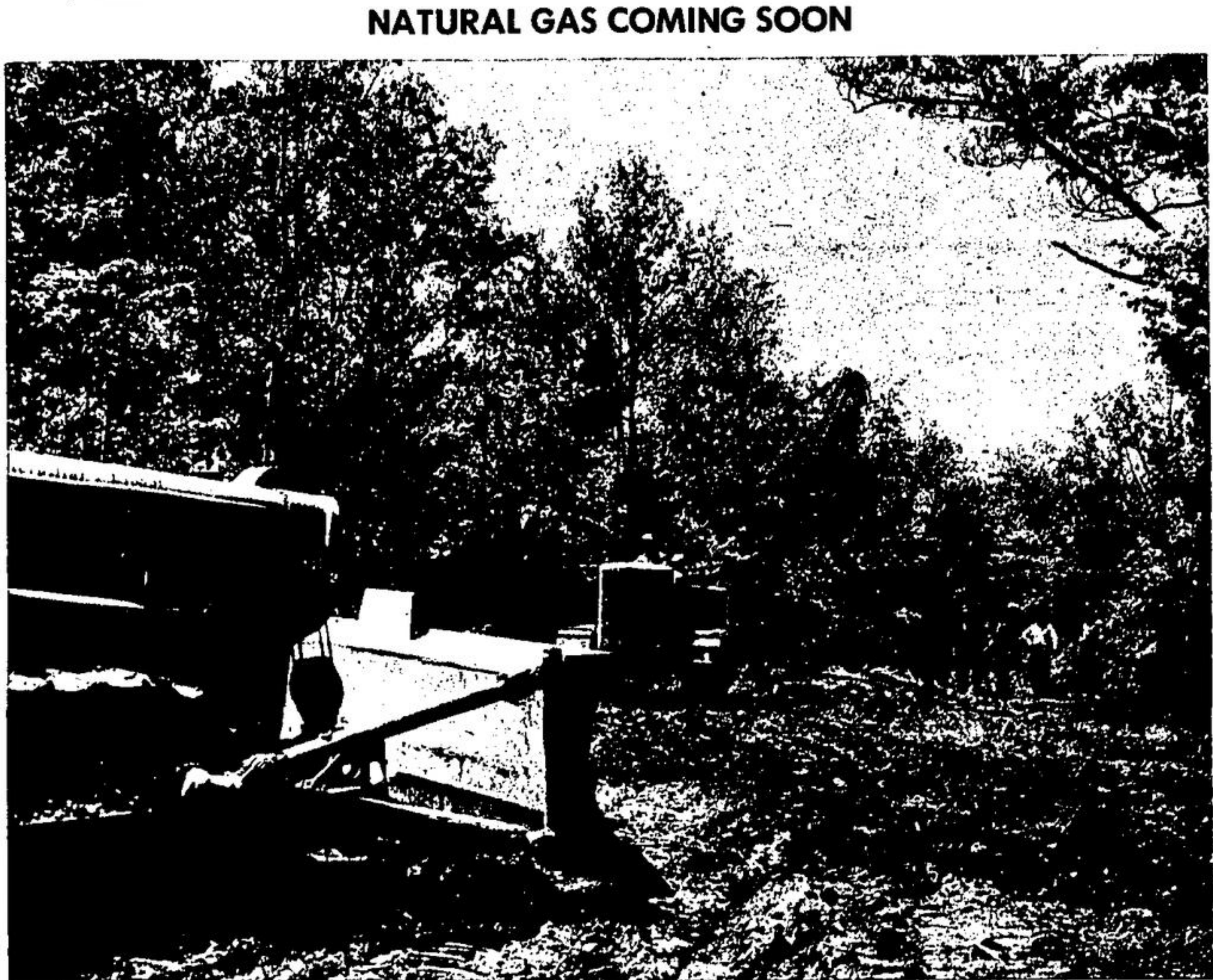
CLEARING THE DENSE UNDERBRUSH is an important part in the preparation for laying the transmission line which will supply Milton, Georgetown and Acton with natural gas. The latest progress report indicates, natural gas will be distributed in the Milton and Georgetown districts about August 1st.
