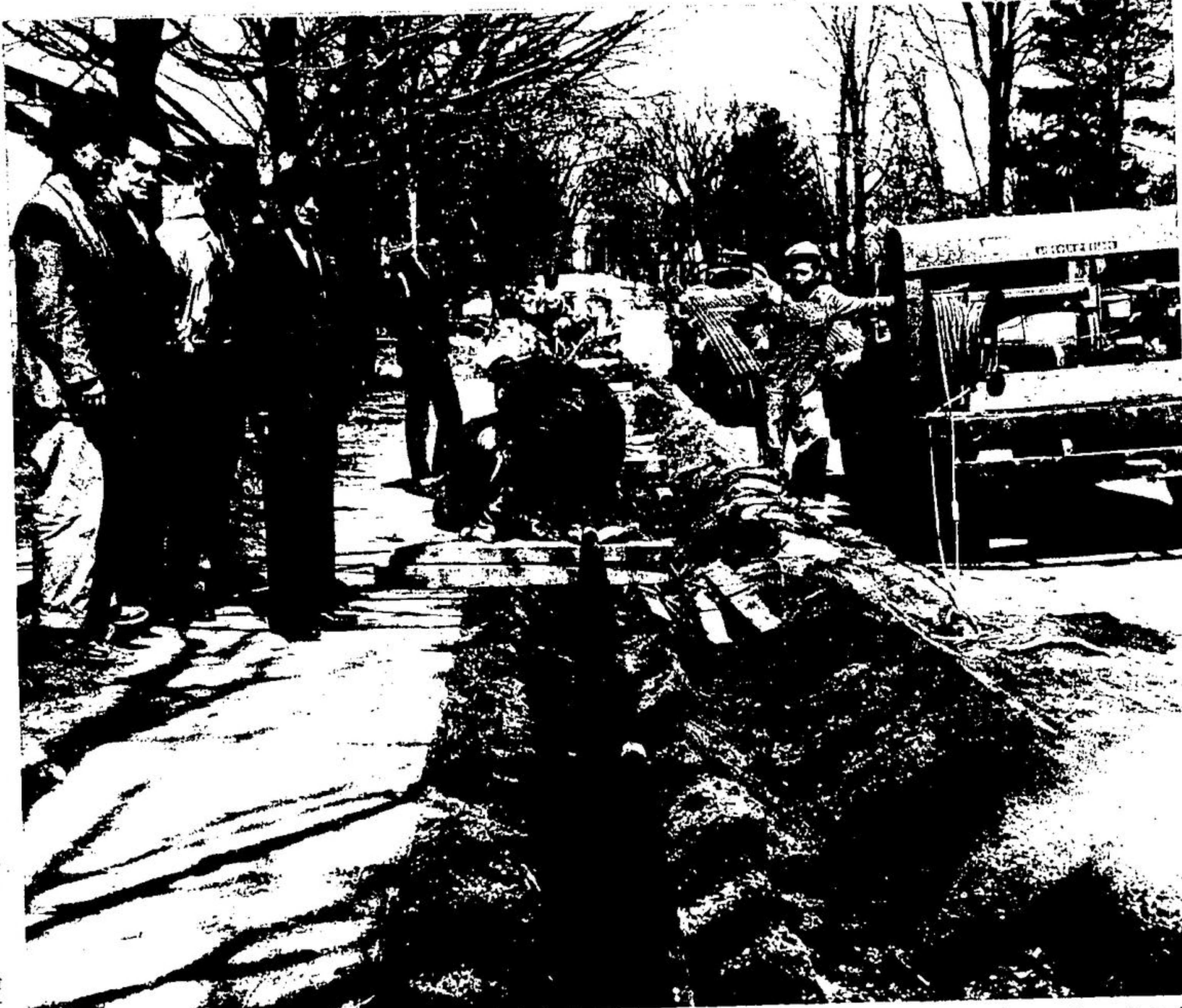
IT'S EASY WHEN YOU KNOW HOW. A group of town officials watch workmen lay the mains which will bring natural gas to Georgetown for the first time in July. On tree-shaded Edith St., where the first lines were laid, pipe is being laid by F. E. Shaw, Ltd., Sarnia for United Suburban Gas Co. Left foreground in picture are town engineer Douglas R. Wilson, Mayor Jack Armstrong, gas company manager Jim Robertson and town clerk John D. Kelly.
