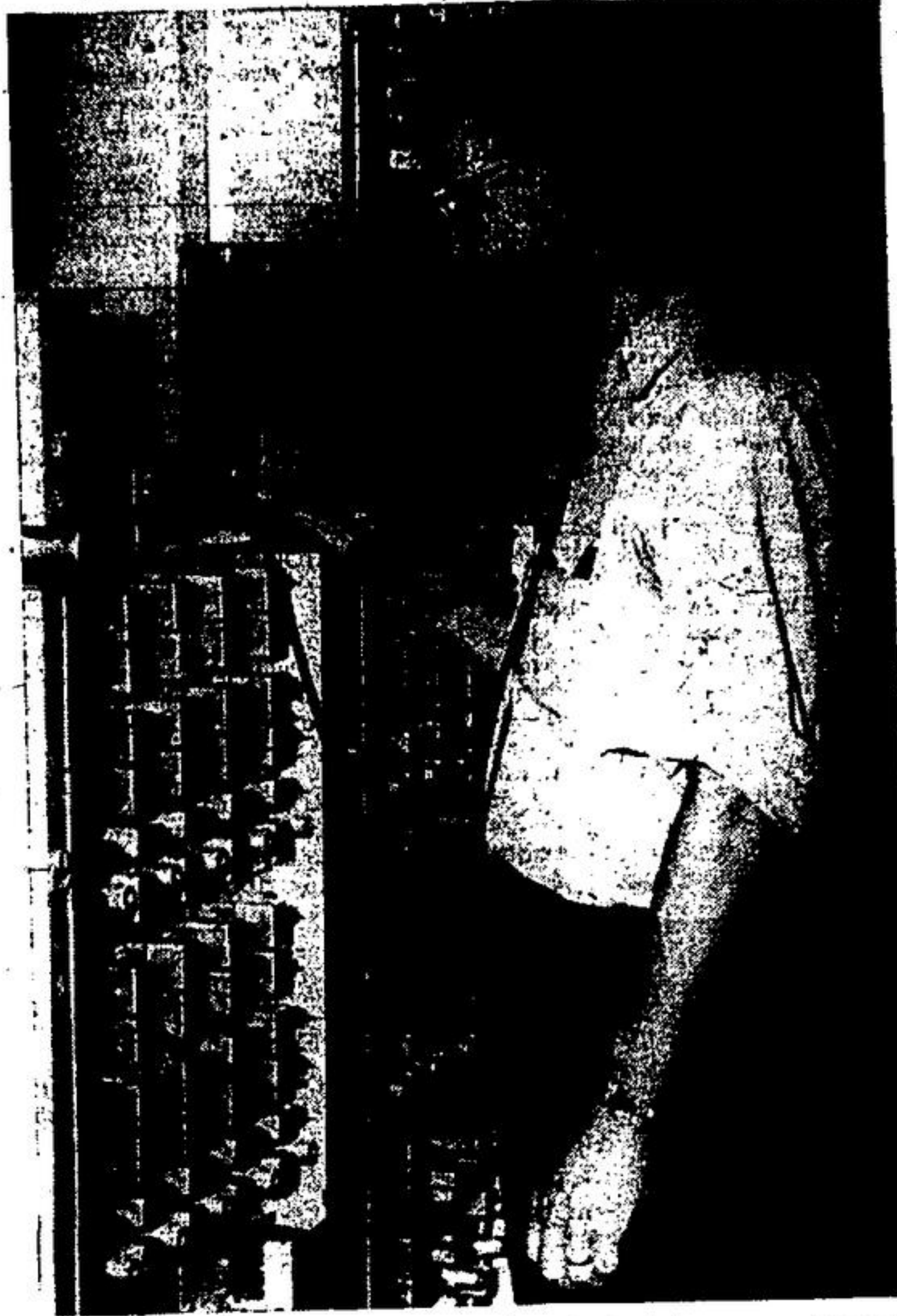
BELL CENTRAL OFFICE MAN Dave Pringle balances up the carriers on the carrier bay in the Georgetown dial exchange. This is the terminating point at the exchange for long distance circuits. It makes it possible to superimpose up to 12 separate circuits on one wire, so that up to a dozen conversations can be carried simultaneously on a single wire.
