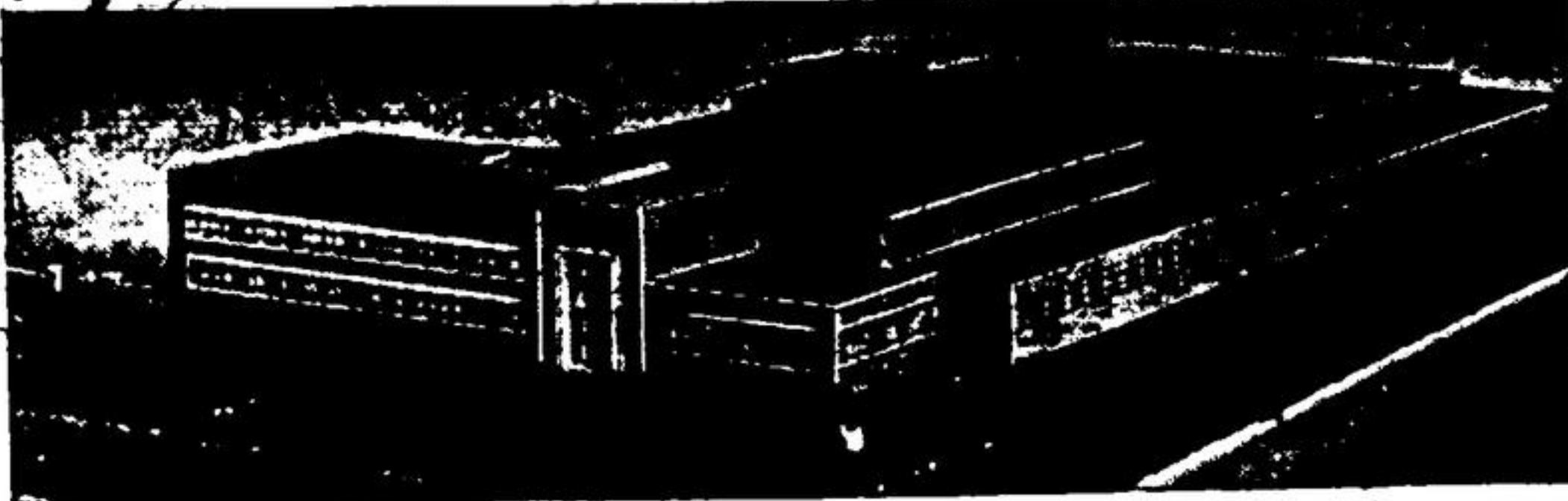
This is the new "SALADA" Tea Building now being erected on Cote de Liesse Road in the Town of Mount Royal, Quebec. It will have a floor space of 125,000 square feet and will feature the modern innovation in North America of blending, packing and shipping on one floor. The building will be completed in 1952, the year which marks the 60th anniversary of the Salada Company and will serve Eastern and part of Central Canada. The other "SALADA" buildings are in Toronto and Boston.
