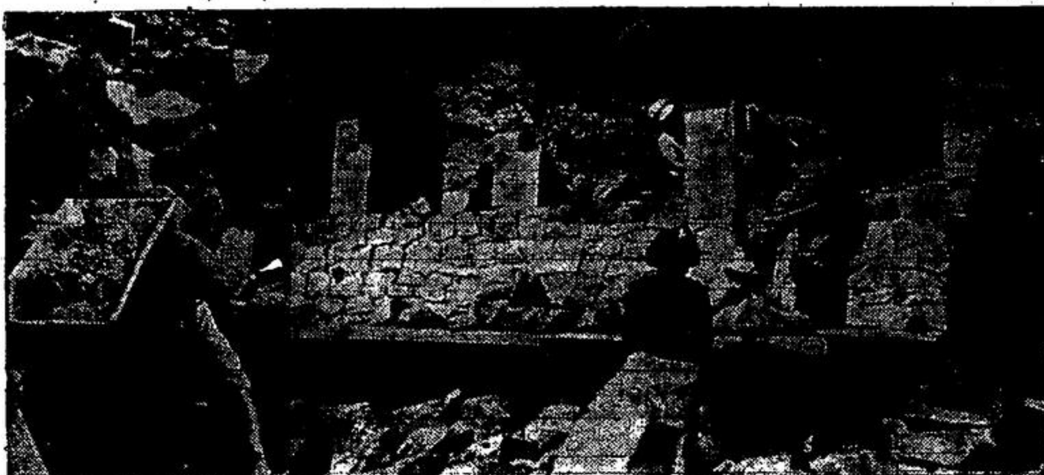
The Greek village of Agnadero had no school. As in many other places its schoolhouse was destroyed during the war. Today, thanks to the contributions of Danish school children and of a team of Danish workers, a new schoolhouse is beginning to rise in the war ravaged Greek town. The initiative was taken by the Danish Society for Reconstruction in War-Ravaged Countries and the Danish National Commission for Unesco. Members of the Danish voluntary team cut stone and mix batches of mortar for the brand-new school which is expected to open some time this summer.
