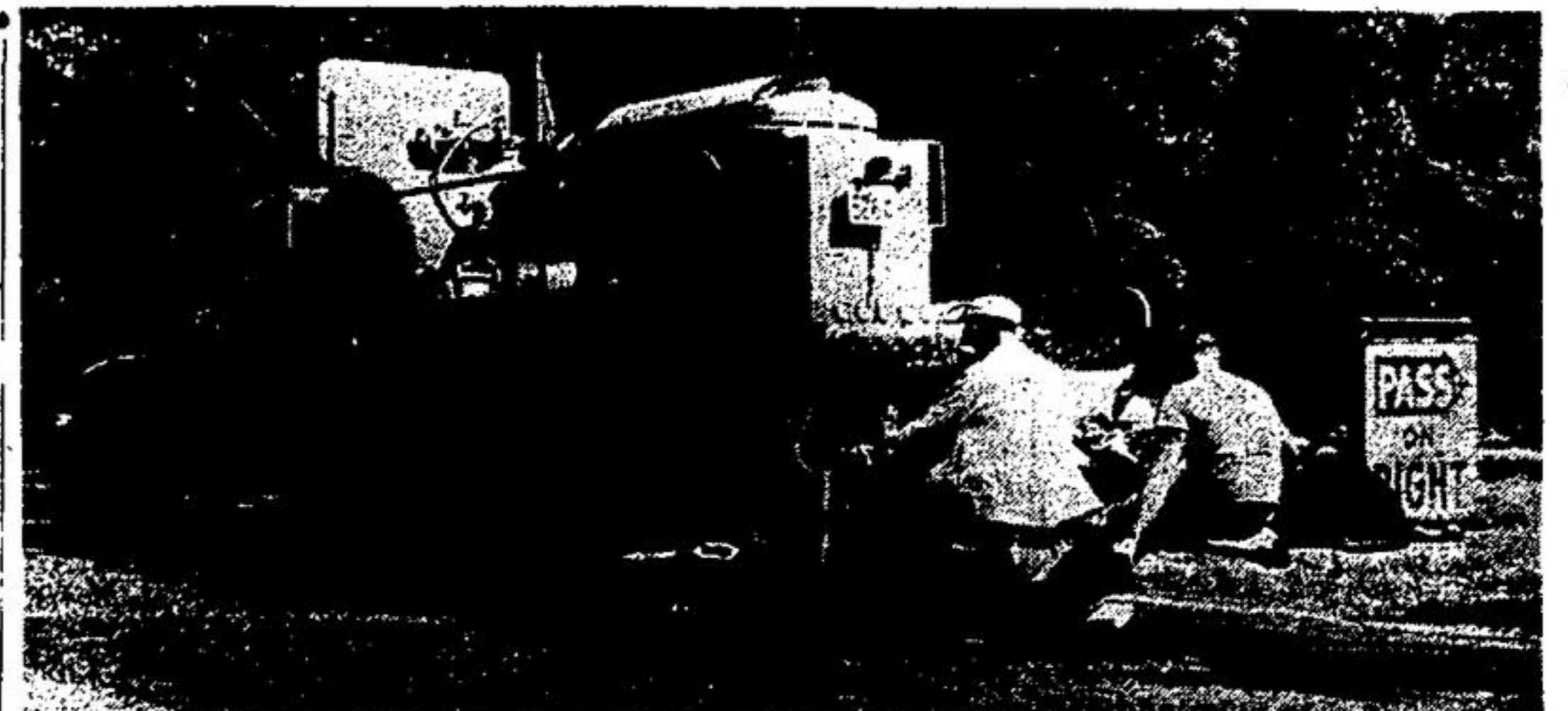
Operator Bruce Dure is ready to pull trigger of spray gun that paints white markings on Ontario highways. His helper, Frank Brewster, is prepared to drop line of red flags warning motorists to keep off the fresh paint. Pointer in front of truck enables driver Ralph Lee to keep operator's gun in the exact centre of road. Ontario Department of Highways operates five of these trucks and so far this year has "white-lined" about 1,500 miles of black highway.
