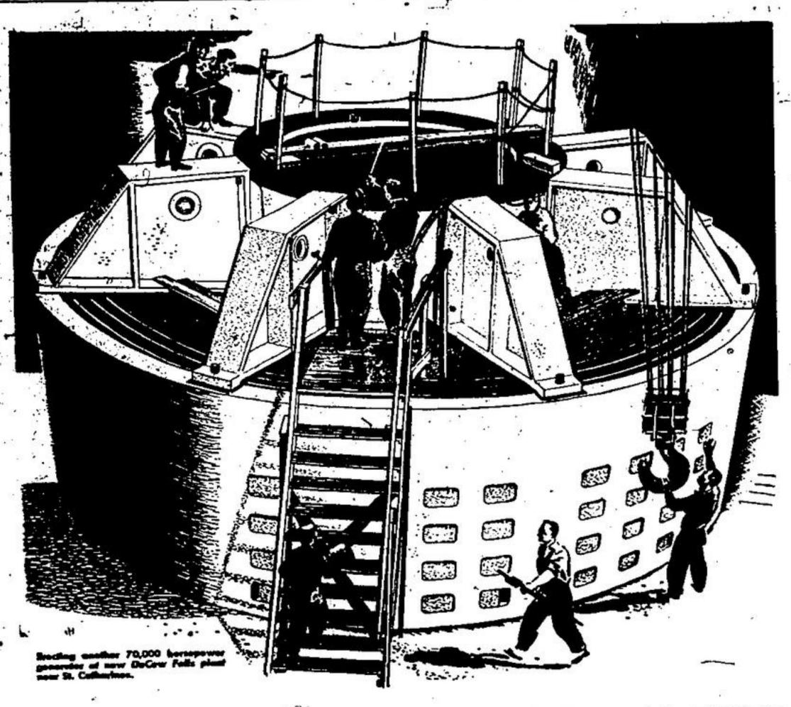
Hydro is pushing construction to meet the pressing demand for more electricity. The above huge generator will soon pour an additional 70,000 horsepower into the Hydro system from the DeCew Falls plant near St. Catharines.
