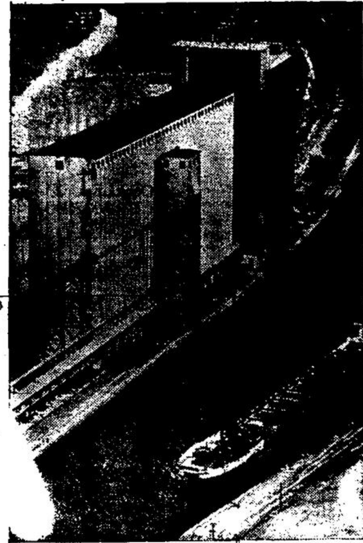
The Robin Hood Flour Mill on the bank of the Welland Canal to which a new million dollar unit has been added to mill cake and pastry flour from Ontario soft wheat.
