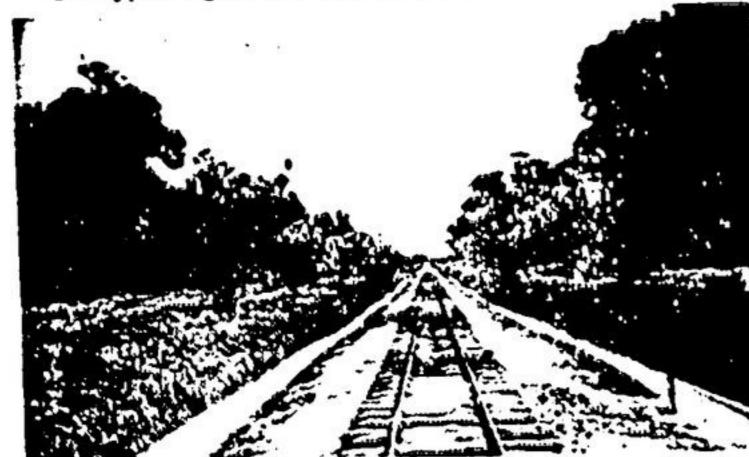
born engineers have just completed constructing a railroad through forty miles of steaming jungle in British Guiana, and they had first to kick the snakes out of the way and then lay the roadbed over and over again because the gravel kept di-appearing into the swamp," says F. L. Parsons, general manager of the Demarara Bauxite Company, Ltd., who oversaw the job.
