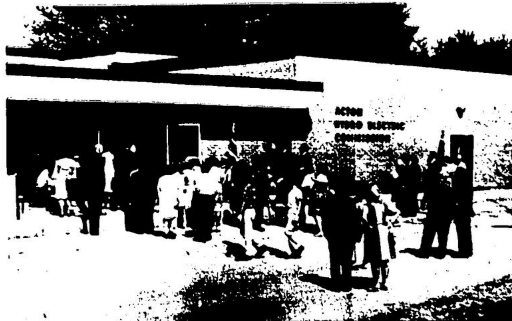
HYDRO BUILDING was officially opened the same day as the centennial library with speeches and a tour for the public.
