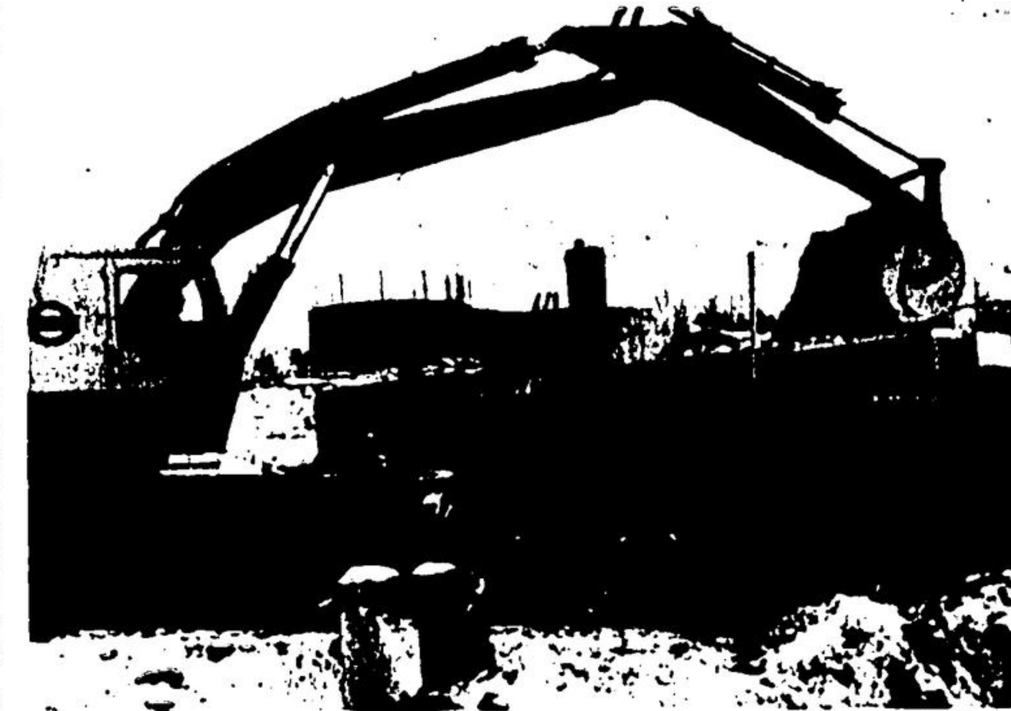
WORK ON THE addition to the water pollution control plant is continuing despite deep snow and frigid weather. Clairson Construction has the contract.—(Staff Photo)
