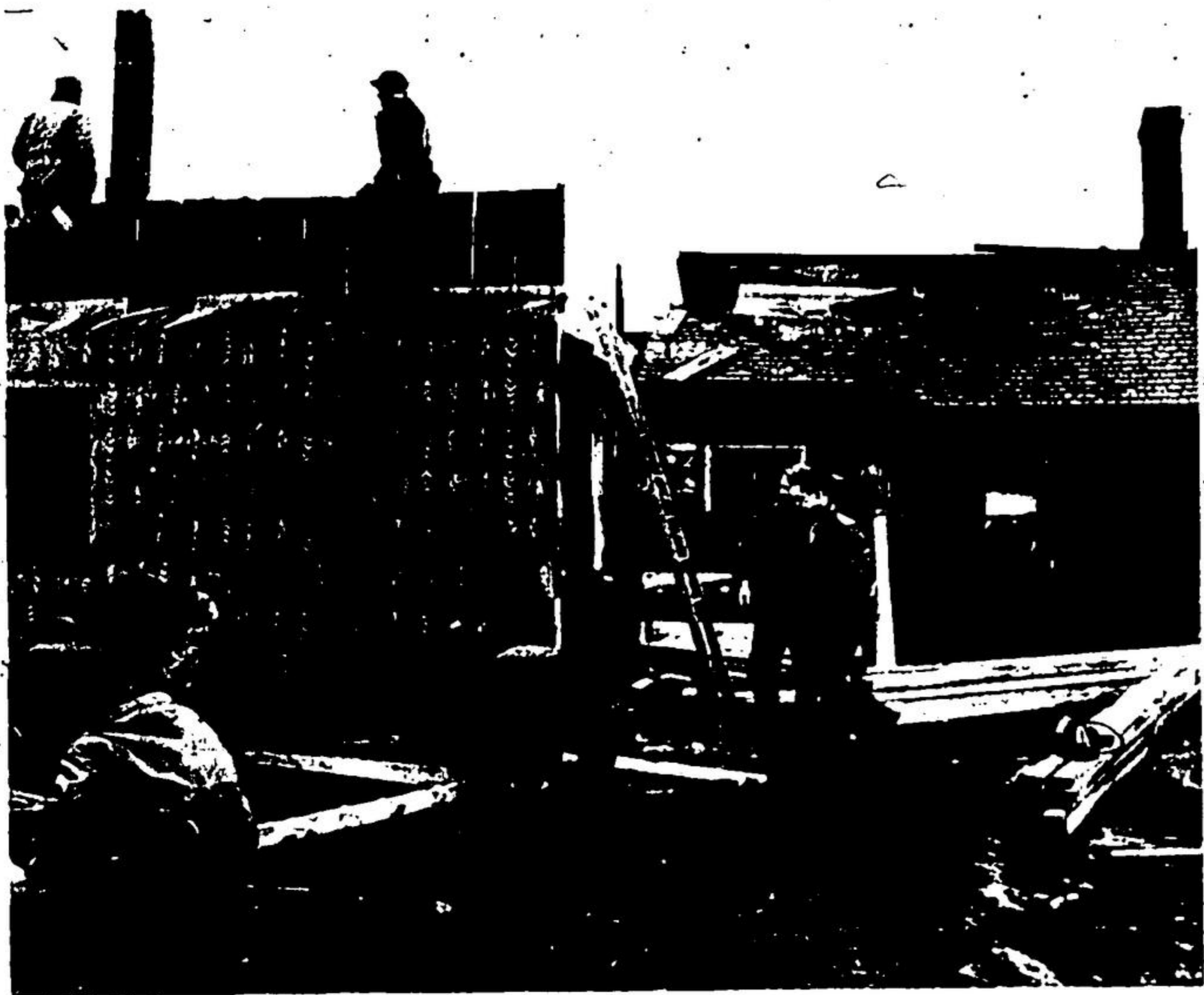
THE SPIRIT OF NASSAGAWEYA and vicinity was evident Saturday as dozens of men converged on the Sixth Line site of the recently burned out home of Mr. and Mrs. M. Bonus and family. The reconstructed building is well on in progress by mid-afternoon. The house was habitable by evening. (Staff Photo)
