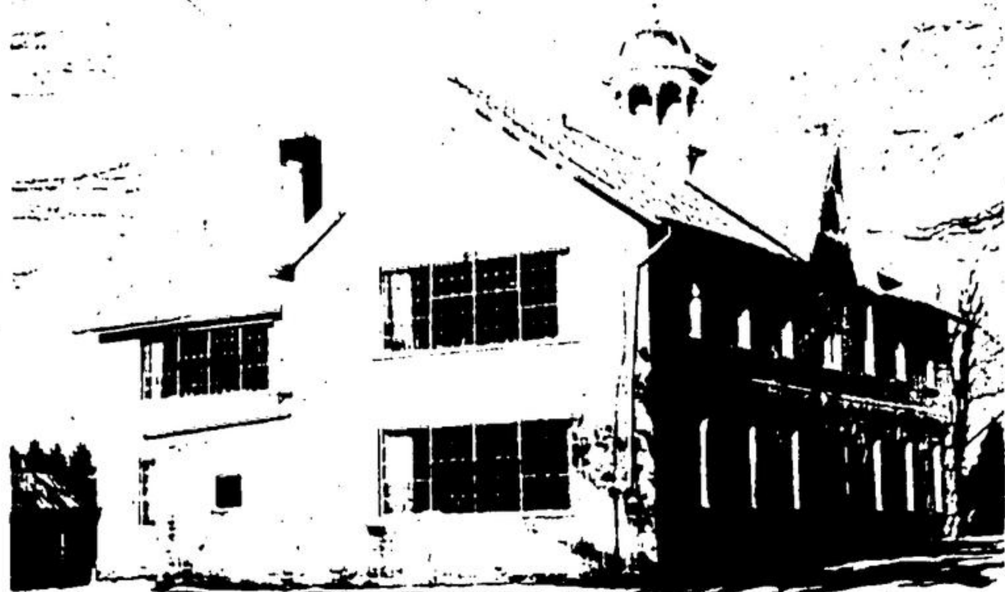
COMPLETED, the Rockwood school was a school bell striking landmark, its cupola housing the old
