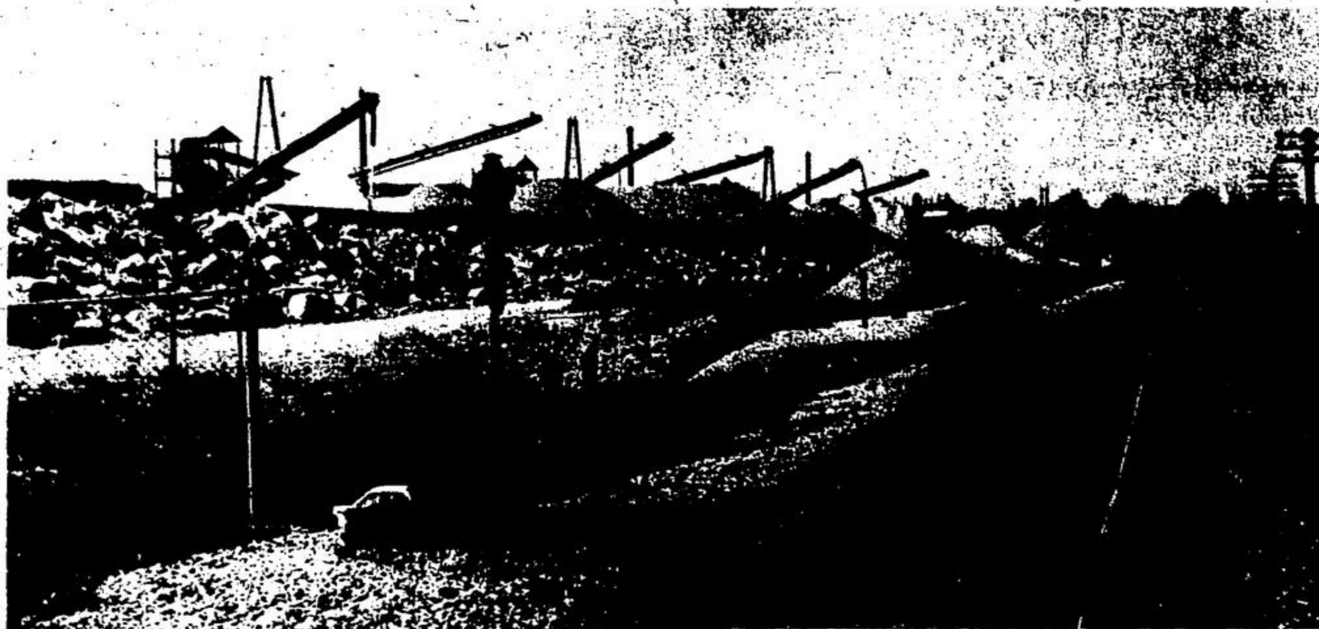
LIKE HUGE FIRING PIECES jutting from behind emplacements, the stone and gravel elevators at Acton Limestone Quarries pile their loads in cone-shaped mounds while railway cars await loads for delivery to building projects. A hive of activity during spring and summer the huge quarry, one of or the largest in Canada contrasts with its pastoral setting between the third and fourth lines.
