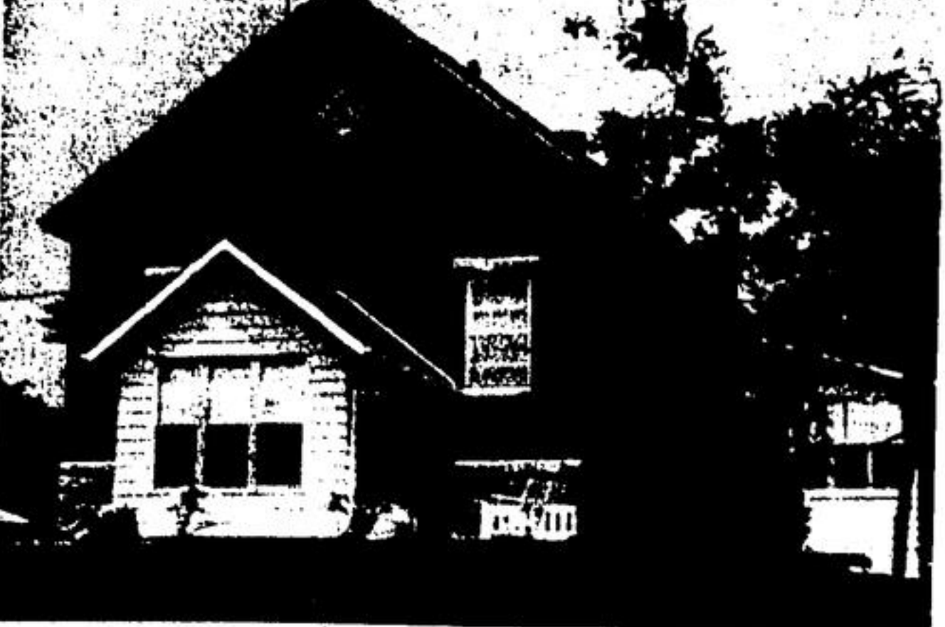
School Now Residence of Dr. Reid
