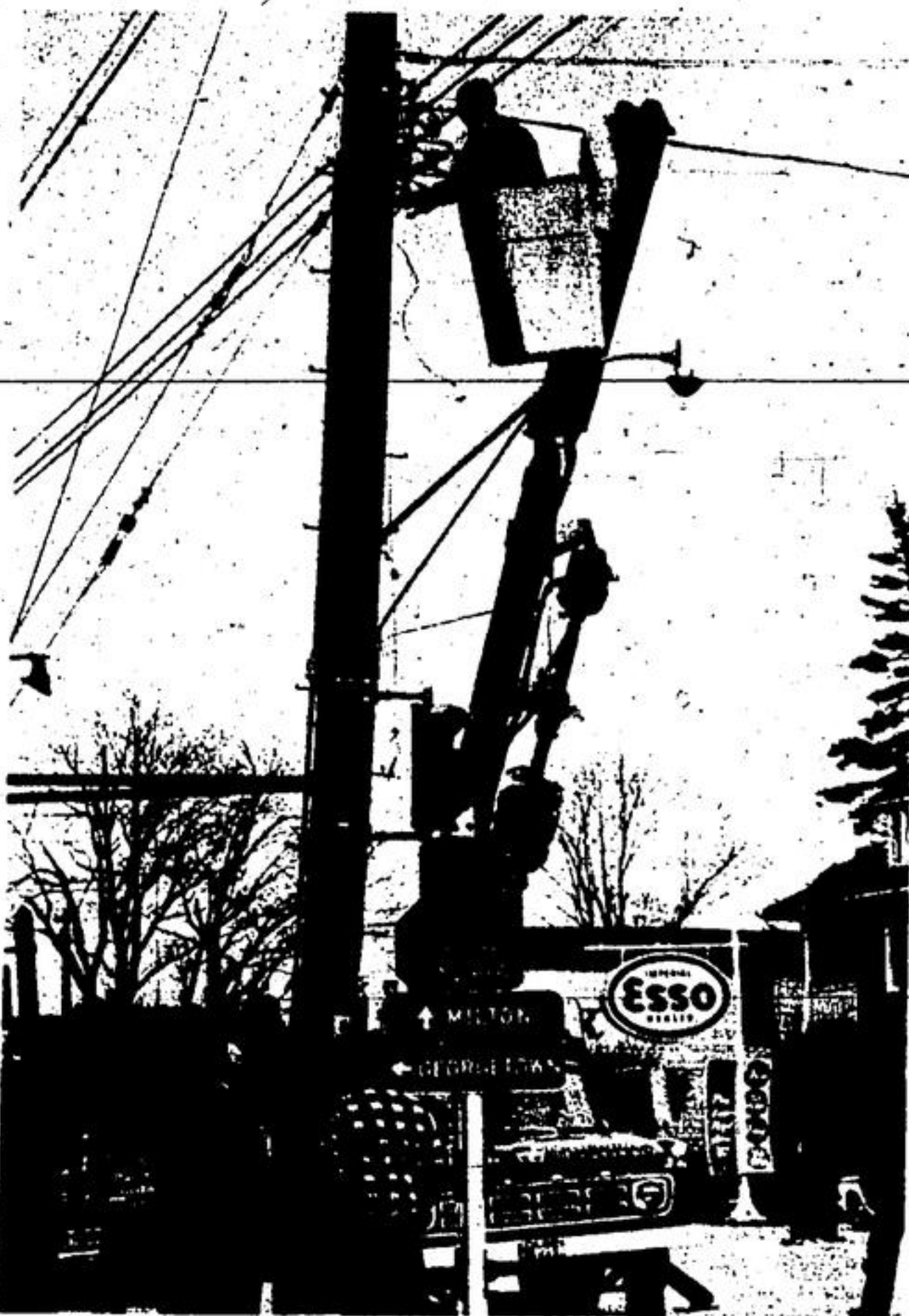
FINAL ADJUSTMENT to wiring is made by hydro linemen Dorson Frizzell as the new traffic lights at the corner of Mill and Main Sts. were turned on Monday morning at 9 a.m. There were no hitches and traffic was soon operating normally. During abnormally heavy traffic the lights can be operated manually at the discretion of a police officer. (Staff Photo)
