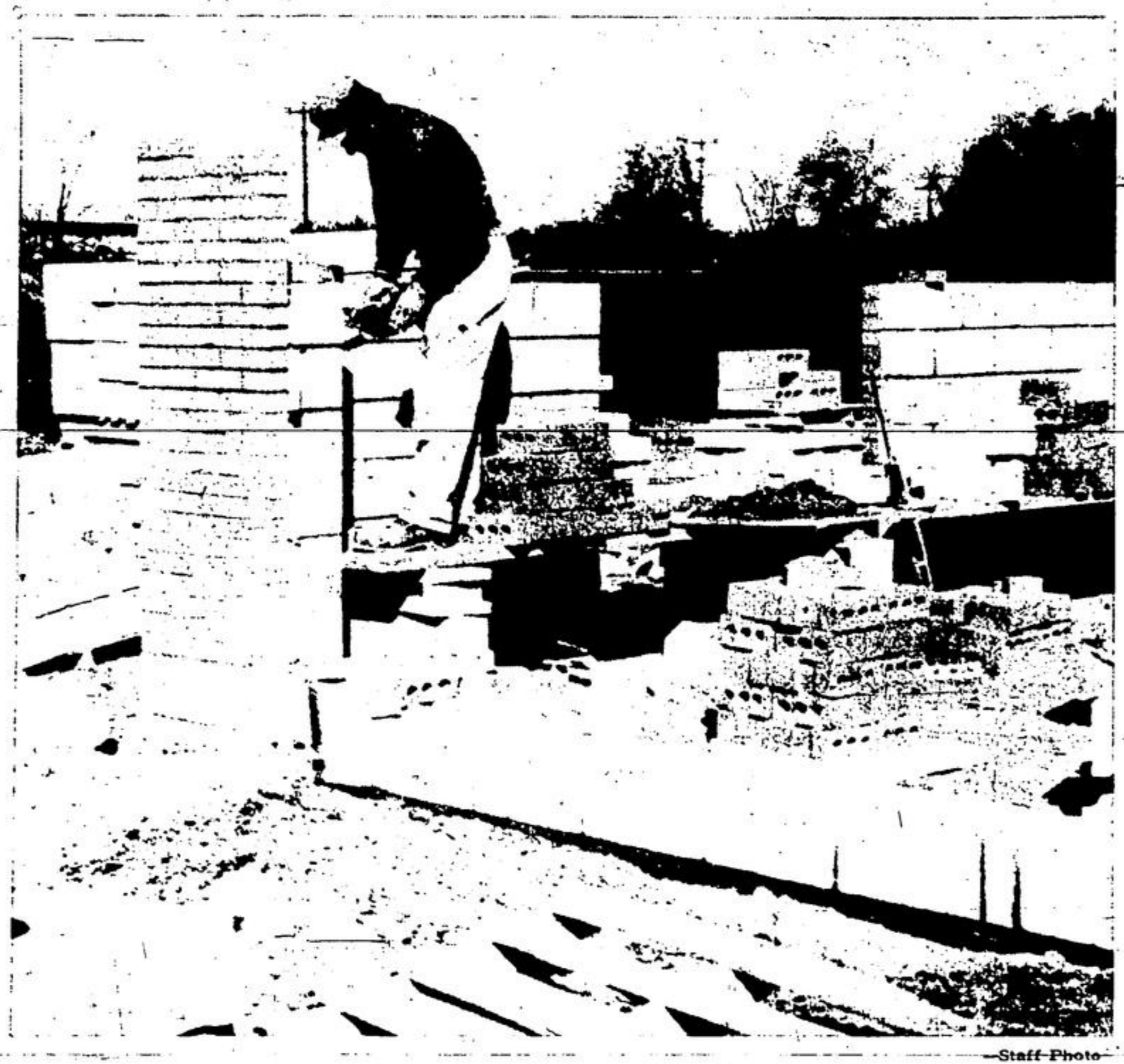
MASONRY CONTRACTORS at work at the site of the new hydro building on Alice Street have been favored with good weather to date. If weather continues in their favor for another couple of weeks it is expected the building will be closed in to allow interior work.
