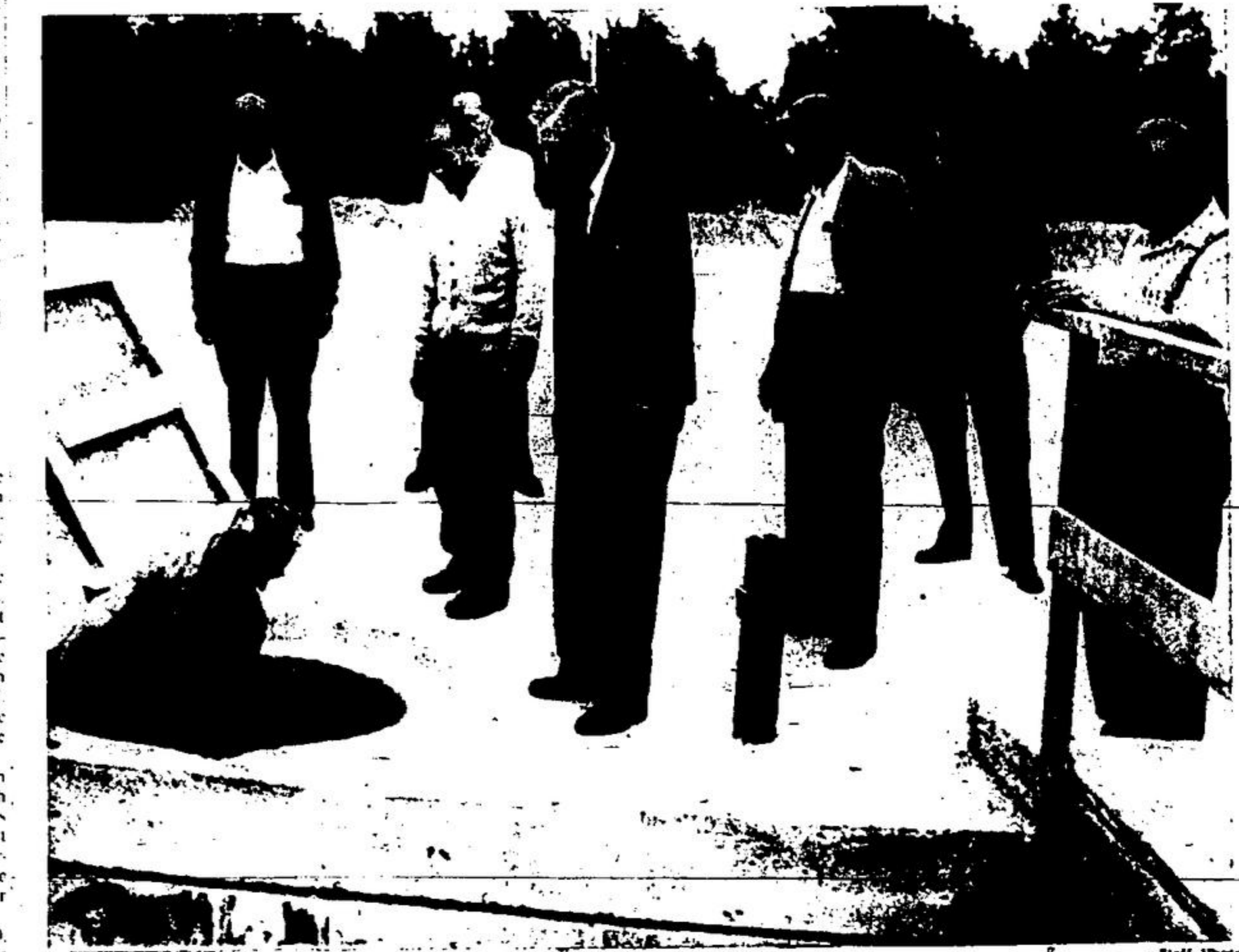
DOWN THE HATCH goes water and sewer chairman Bert Wood during the Council's inspection tour of the new water reservoirs seen in the picture are Mayor John Goey, Reeve Jack Hargrave, Deputy Reeve Bill Denny, Councillors Les Doby and Frank Toth, Clerk Jack McGeachie and Assessor Bill Erskine. The two tanks now nearing completion have a diameter of 83 feet and a depth of 15 feet. On the tour and during the Council's inspection tour of the new water reservoirs seen in the picture are Mayor John Goey, Reeve Jack Hargrave, Deputy Reeve Bill Denny, Councillors Les Doby and Frank Toth, Clerk Jack McGeachie and Assessor Bill Erskine. The two tanks now nearing completion have a diameter of 83 feet and a depth of 15 feet.
