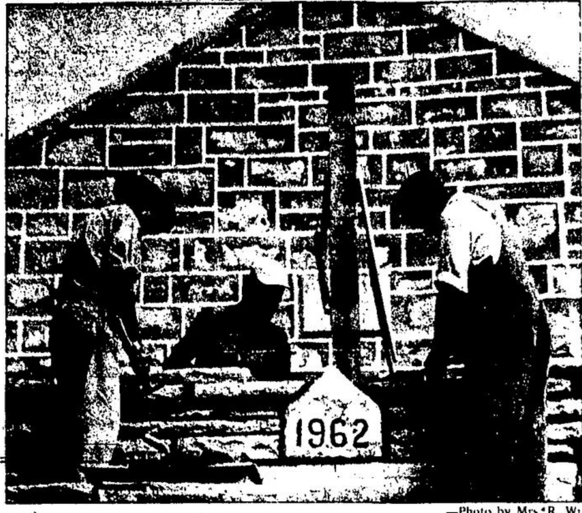
EDENS MILLS United Church is undergoing a facelifting this week along with an extension to the front of the church with Georgetown cut stone. The walls have been tape-pointed and two stain windows added. Workmen pictured above include Reg Rudd, Wilk Wilson and Bob Wright. A new date stone 1962 will be included in the renovations.
