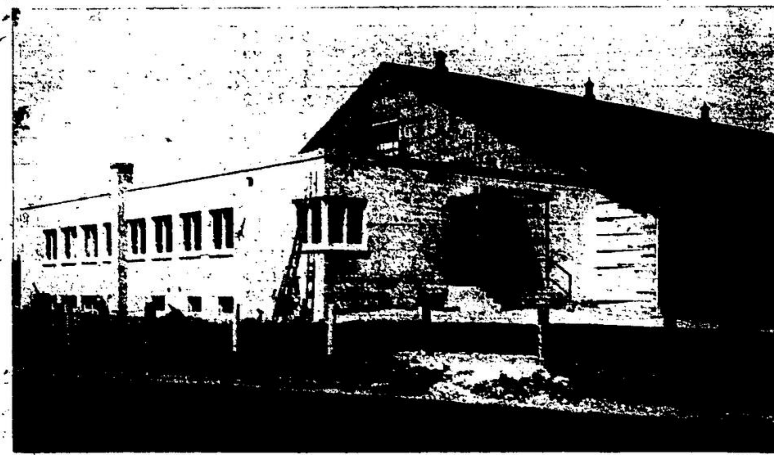
"FINISH IT NOW" VOLUNTEERS will make their house-to-house canvass of Acton homes early in June. The fund raising campaign was launched to clear the deficit on the building program and to complete the project with the finishing touches. When the canvasser calls at your home you will be asked to continue your pledge for an additional two months, if you are contributing on
