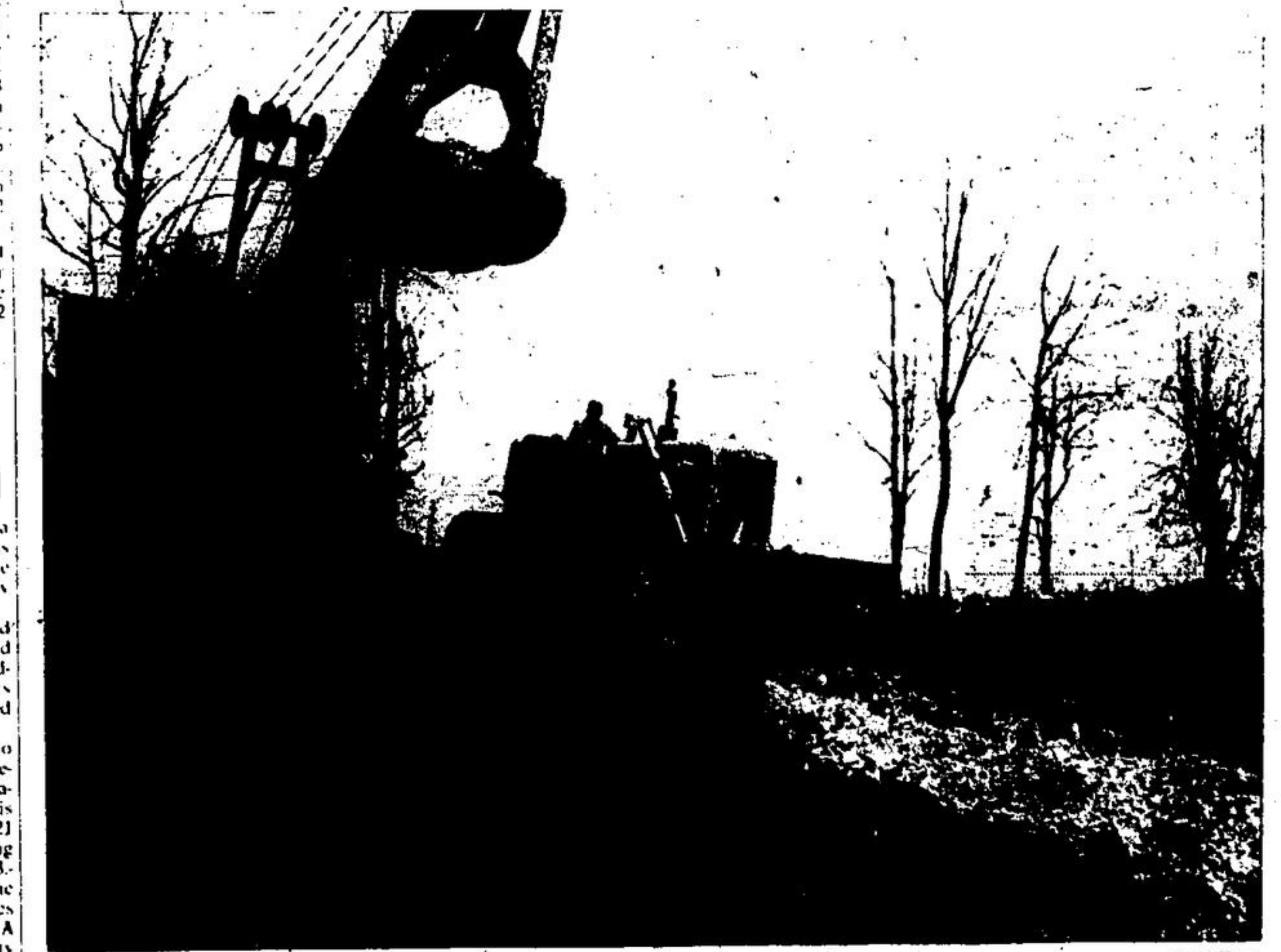
EXCAVATION STARTED for the new water reservoir being expected to have the excavation completed by next Wednesday, built on Churchill Road North this week and power shovel. When this phase of work is completed, footings will be poured, and bulldozer operators have been kept busy. James Kemp Steel has been arriving at the site this week and engineers are on hand to watch the progress.
