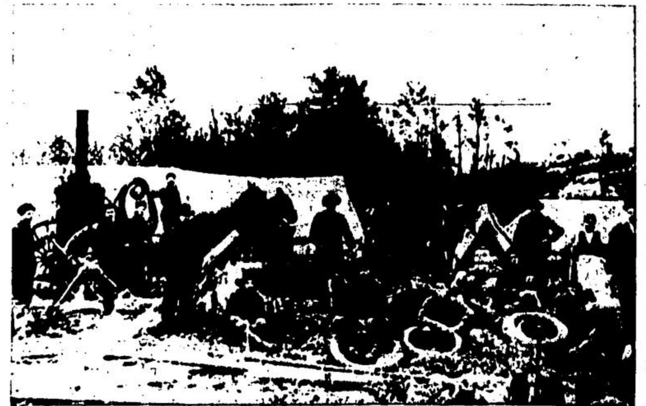
TELEPHONE LINEMEN building Acton's first line camped out along the way. This telephone crew of the 1900's is complete with moustachioed cook and bearded blacksmith. Note the horse-drawn steam boiler for power for pumping and drilling.
