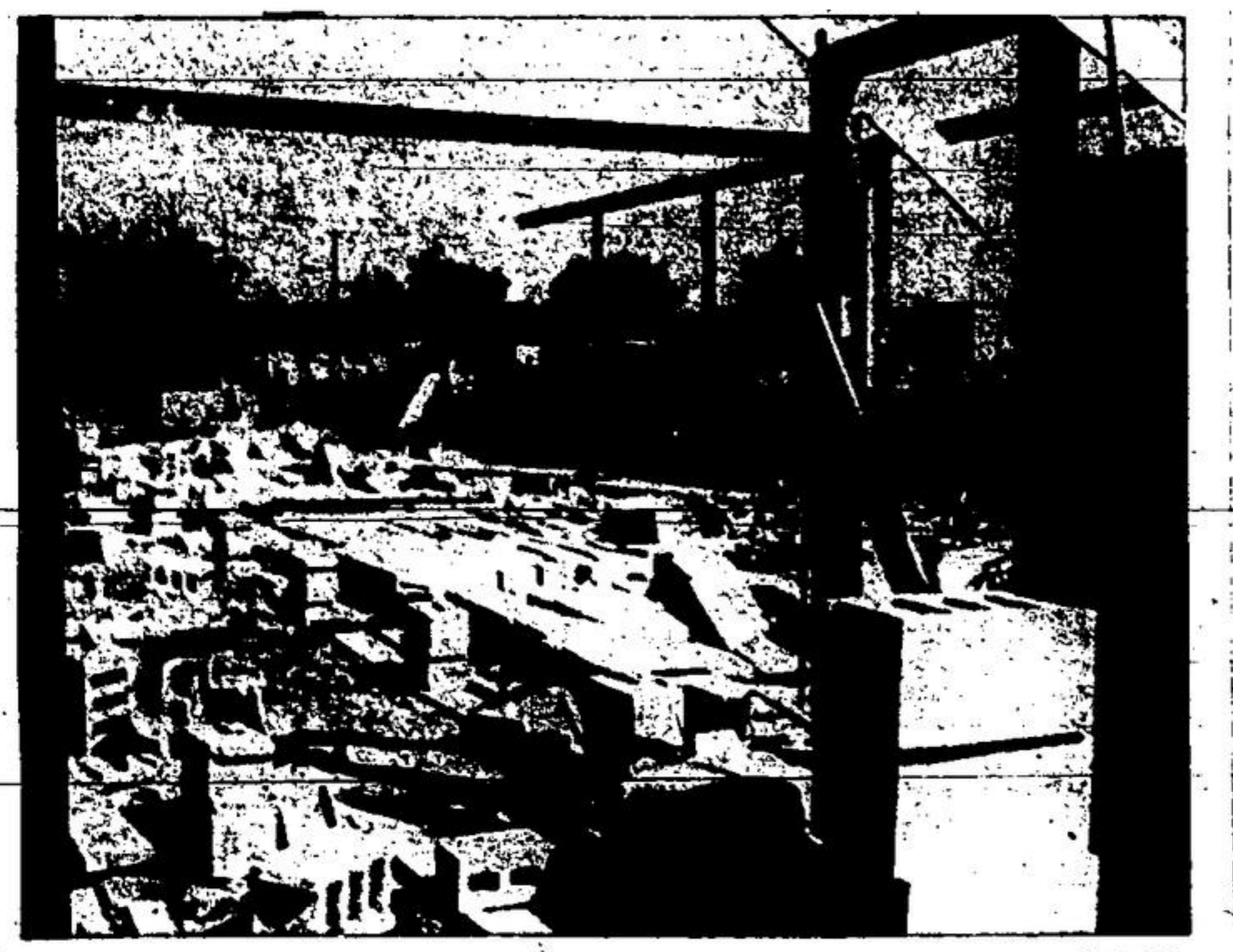
—Staff Photo THREE-DAY SETBACK in the construction of the new central school at Brookville was caused when high winds during a storm knocked down a corridor wall last Friday. Workmen had just completed the wall before finishing for the day when the storm struck. Some of the cement blocks are specially glazed and costly and it is believed that of the 900 blocks affected, all are damaged beyond further use. It is also believed that plumbing, wiring and door frames are smashed and will have to be replaced. The above photo shows the section of the wall which collapsed.
