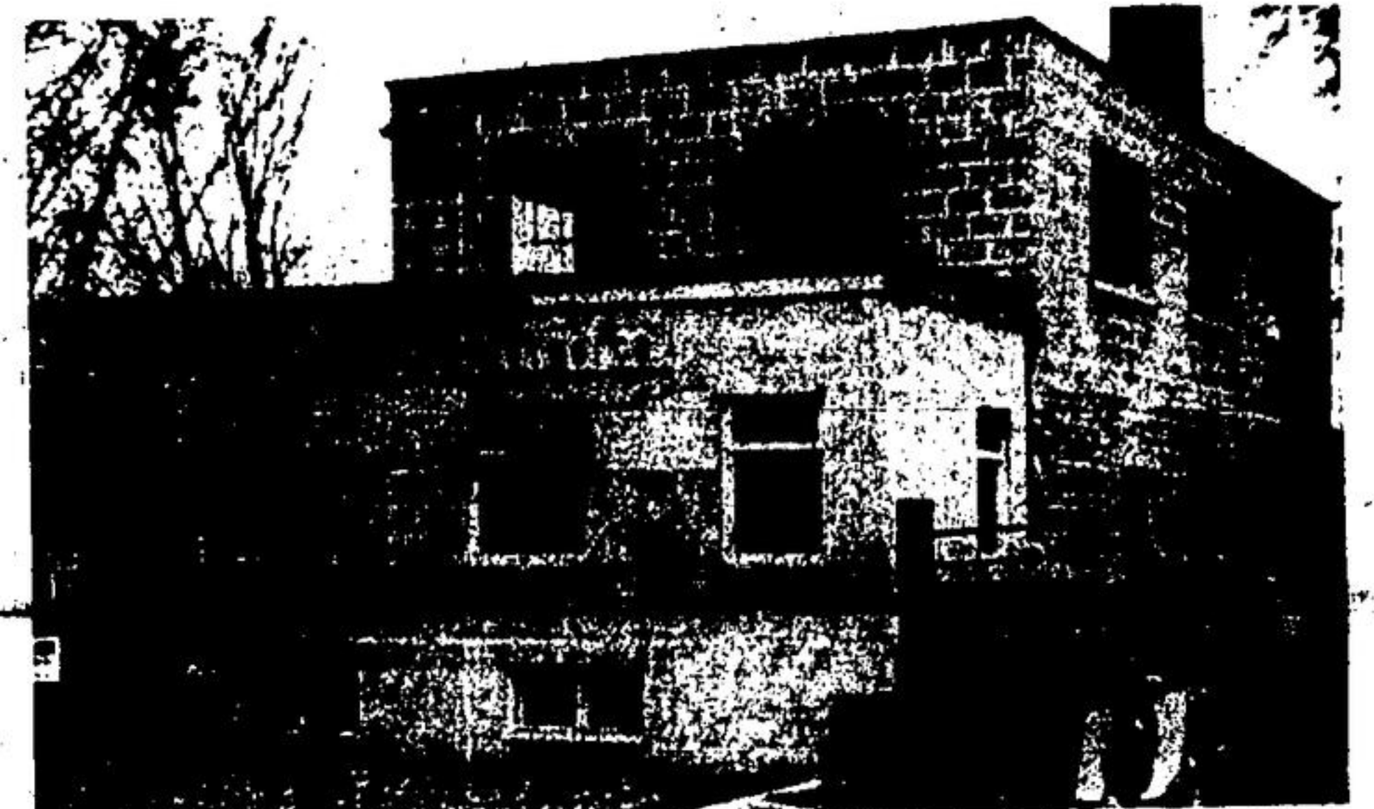
Formerly the Mason Knitting Co. building, the Baxter plant has since been enlarged. This view was in 1940.
