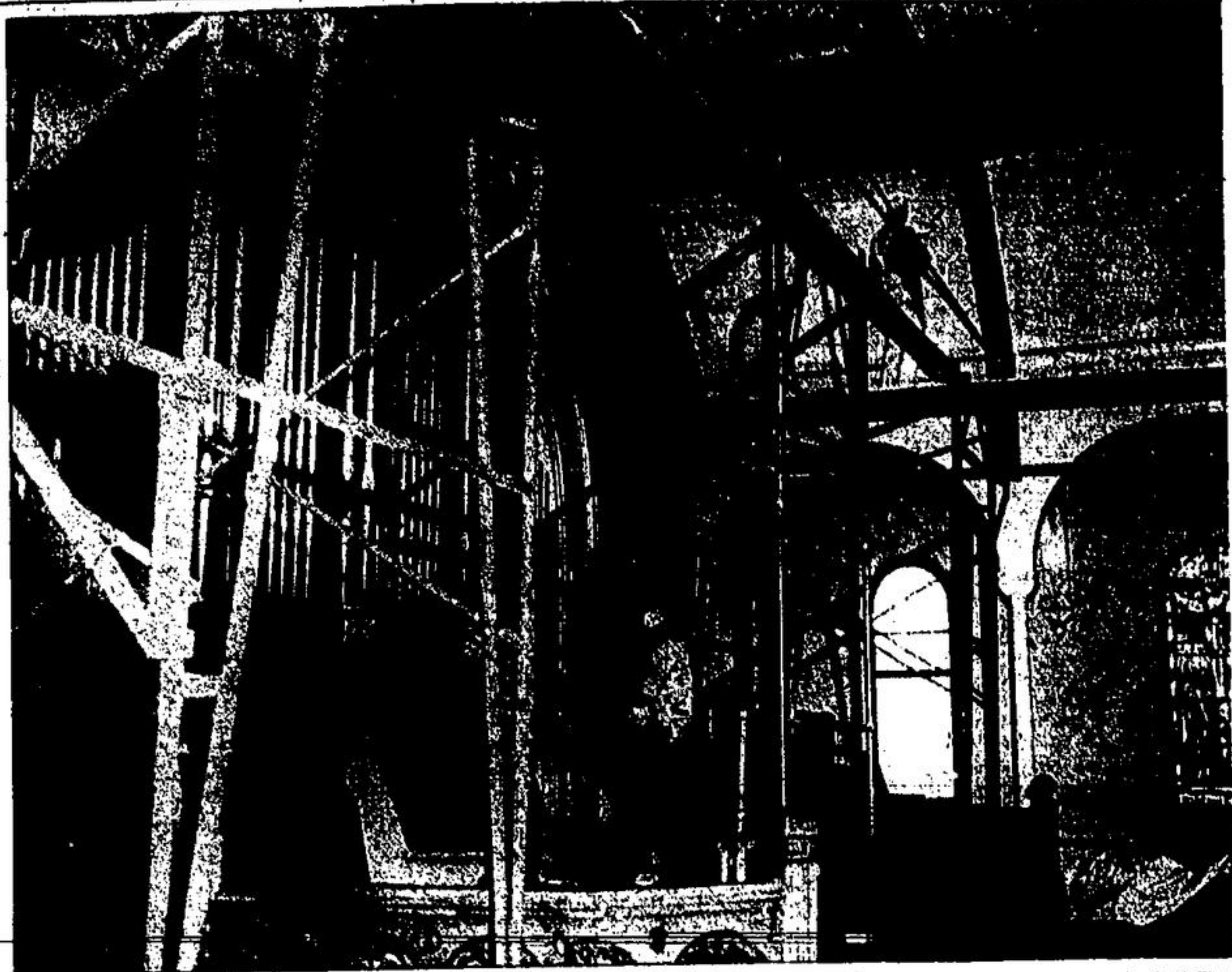
SCAFFOLDING RISES to the ceiling of Knox church as painters are at work in the interior of the building. BOB Frank takes down the hymn board while Tony Frank and L. Slingerland paint, standing on boards supported by the sturdy steel frame. Pews were not removed for the task, but the congregation joined in services at Acton United Church last Sunday.
