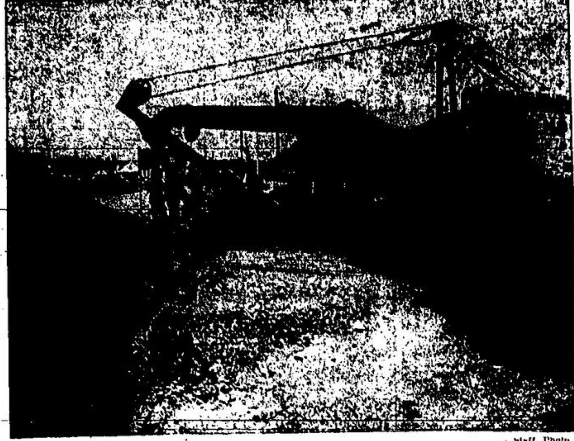
STORM SEWER INSTALLATION is under way in the Glenlea Subdivision in Acton and a huge shovel is pictured above as it scoops mounds of earth out of the roadway as workmen follow close behind laying the sewer pipe. The Durban Construction Company of Toronto is subcontractor for the project and is endeavoring to complete the job as soon as possible before paving is started.
