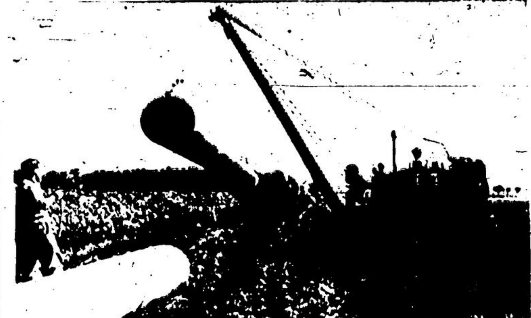
LARGE, 26-INCH PIPE for Union Gas Company's new natural gas pipeline began arriving at the western end of the line on Monday. The line, which will run from the Company's underground storage station in southern Lambton county to a point near Oakville, will supply natural gas to such places as Stratford, St. Mary's, Stratford, Waterloo, Kitchener, Guelph and Hamilton, plus a number of other communities.
