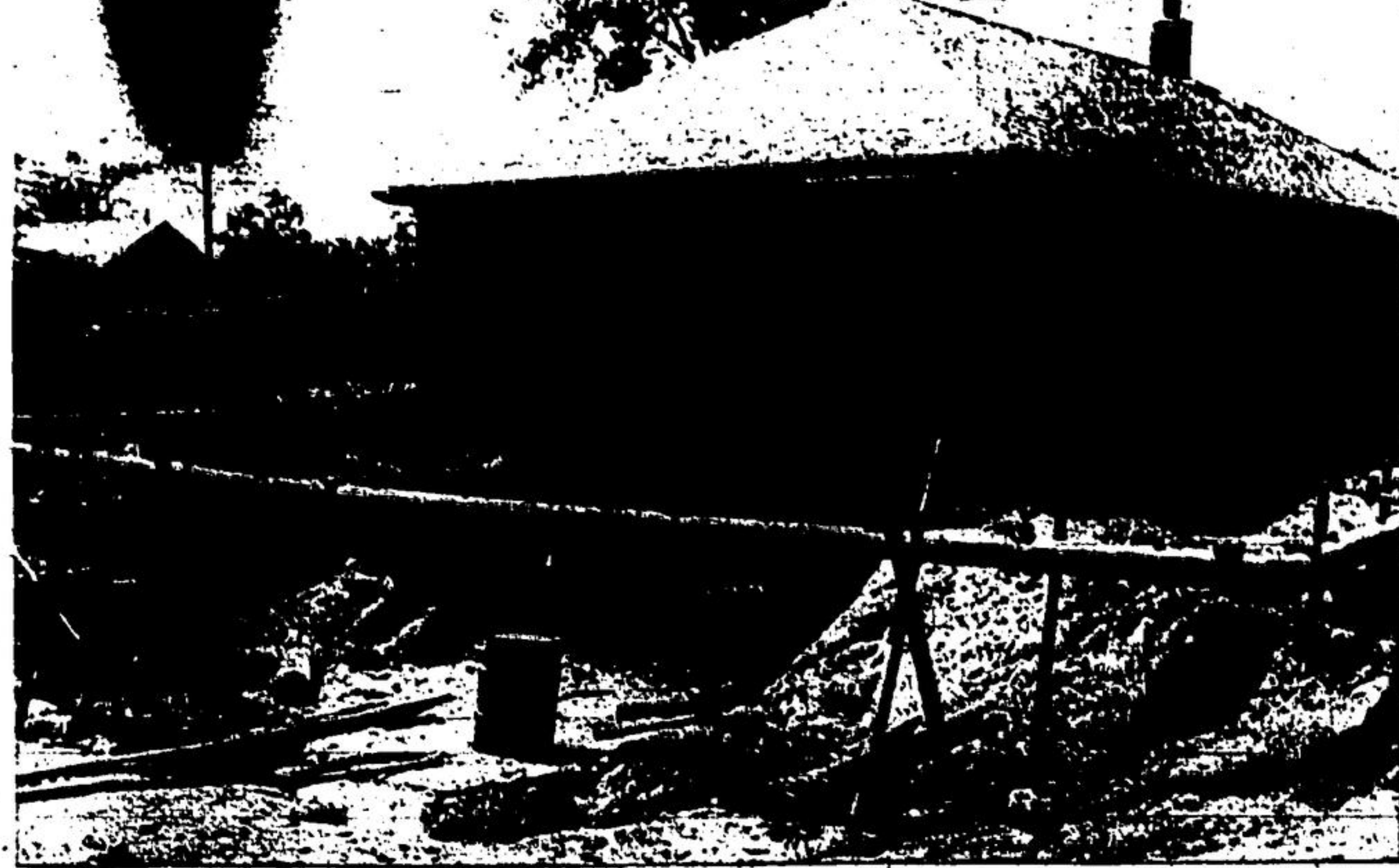
BASEMENT EXCAVATION at the local Scout Hall is now proceeding since the installation of well-points to drain the area and allow digging in the sandy soil. The hall is resting on steel beams supported by posts in the centre and the outside banks.
