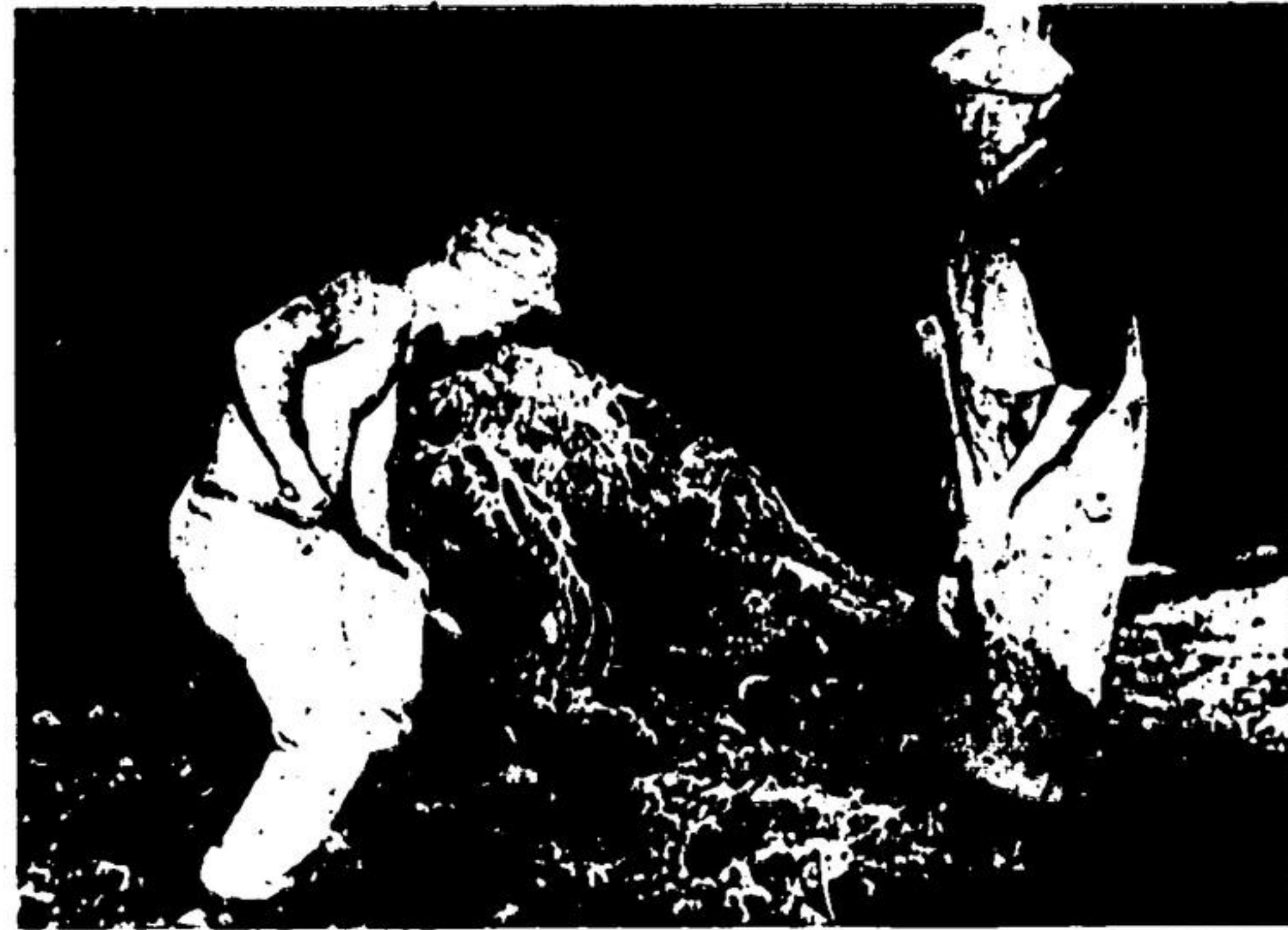
HAND EXCAVATION around the edges for the basement addition at the Scout Hall is being done by Albert Van Gils and Hank Ullterwick. Constant caving in the sandy walls delayed work until well points, to remove the excessive water in the area, were installed.
