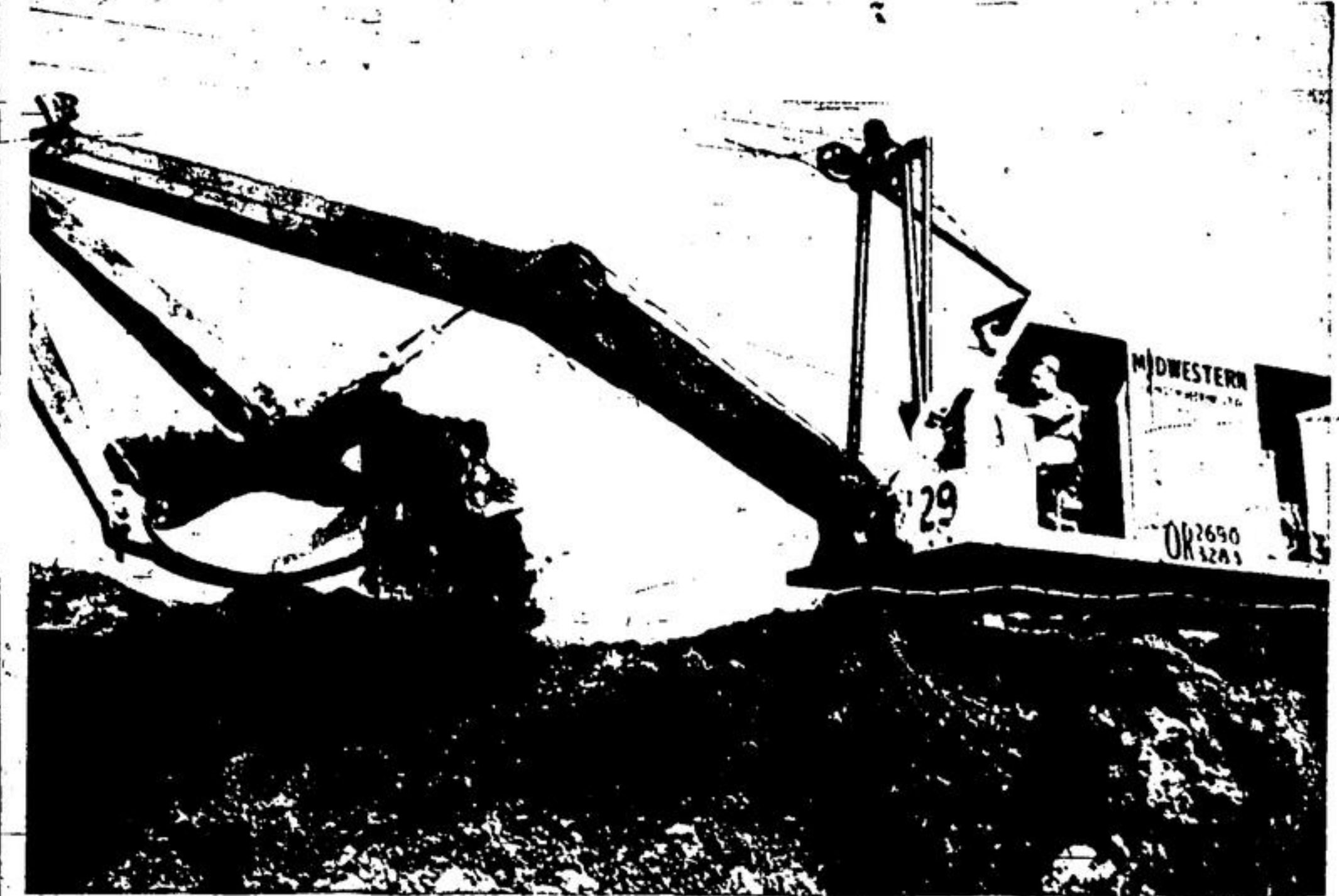
EAST END CONSTRUCTION is typified by this power shovel seen gouging out the foundation for the new Christian Reformed Church. A Pentecostal church was also being planned in October.
