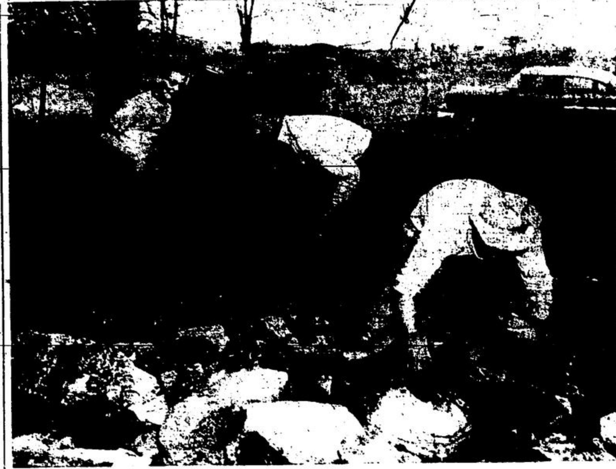
FIRST MOFFAT SCOUT CAMP is being set up on the farm of Scout Master Don Kennedy, north-west of Campbellville, and one of the biggest jobs is building a roadway through the dense swamp leading to the site. Scout Master Kennedy and two of his scouts spread around some of the field stones that have been dumped by tractor to form the foundation for the roadway.
