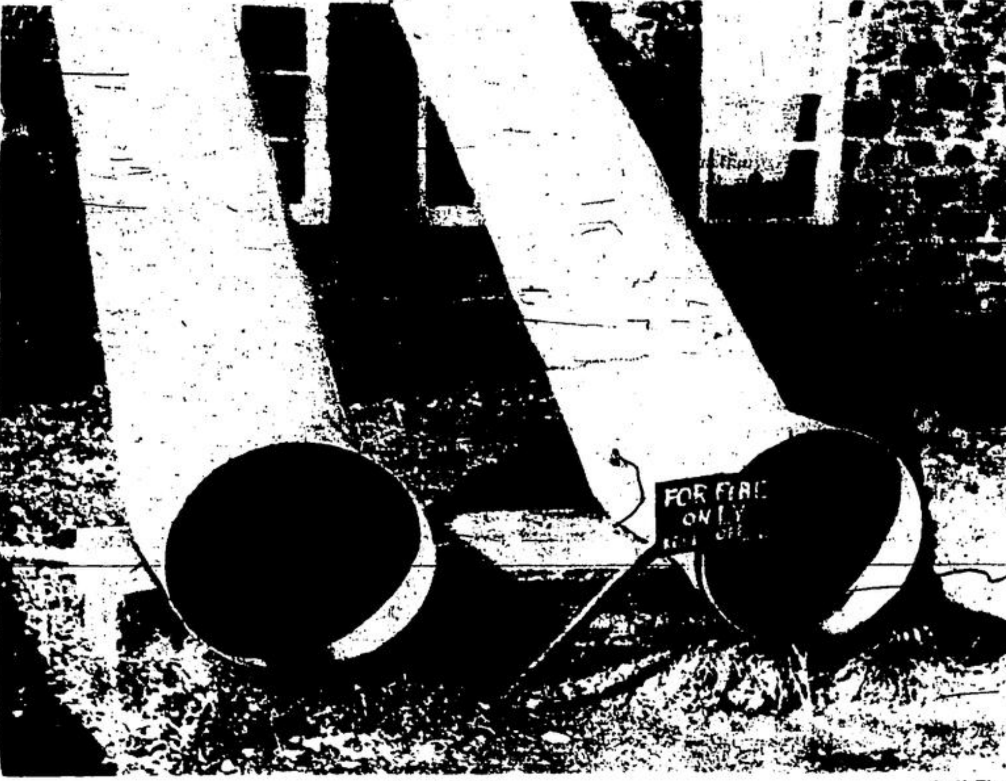
WATER FLOWS FROM ESCAPE chutes on the south side of the burning wing in last week's fire at the Public School. Fortunately, the two chutes weren't needed as the building was nearly empty at the time of the noon-hour blaze. The water spread in a big puddle as it flowed from the roof.
