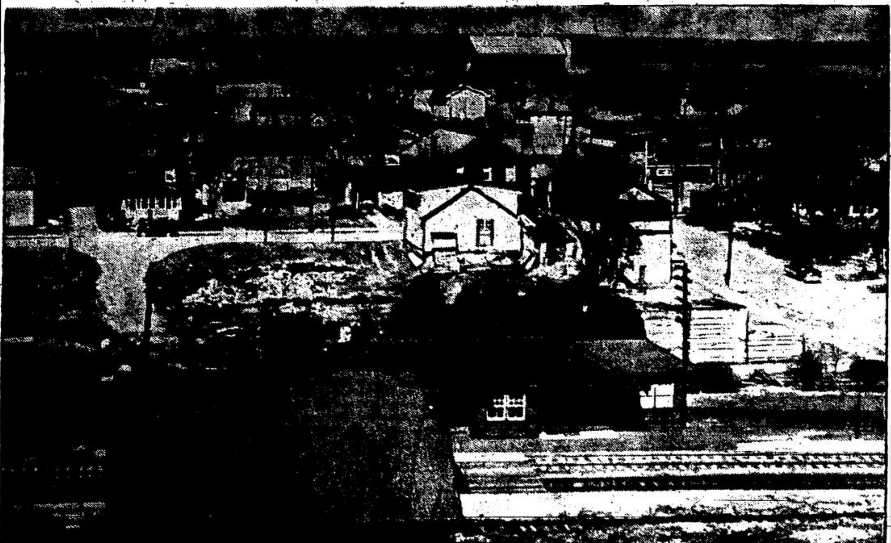
PICTURESQUE CAMPBELLVILLE was the subject of a feature story in recent evening's edition of the Toronto Telegram, and, as shown in this photo which made up part of the feature, the village, though small, could some day be the scene of bustling industry.
