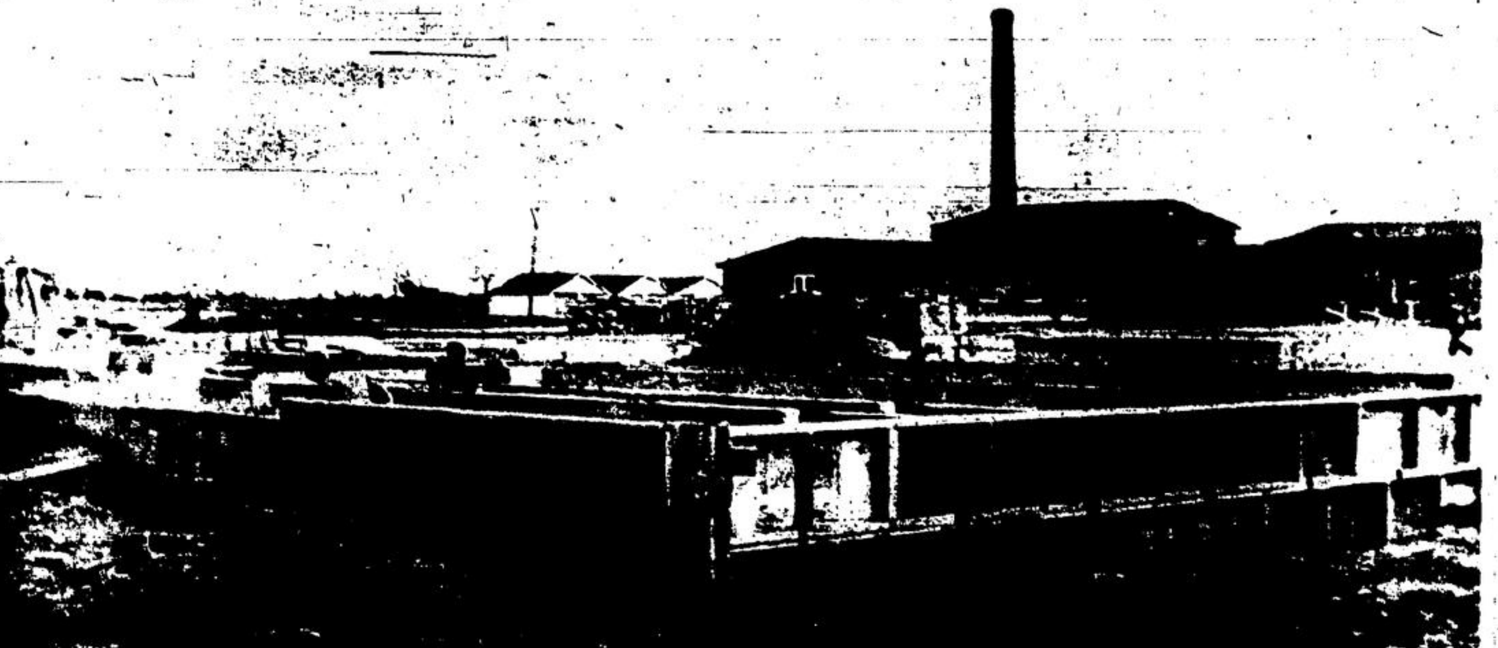
STAFF HOUSE at Halton Centennial Manor, just south of Milton, is now well underway. The foundation has been poured and work is continuing with the good weather. The new house, which will accommodate the Manor staff is situated just north of the Manor buildings, seen in the background at the right. Estimated cost of the new building is about $115,000 which includes interior furnishings.
