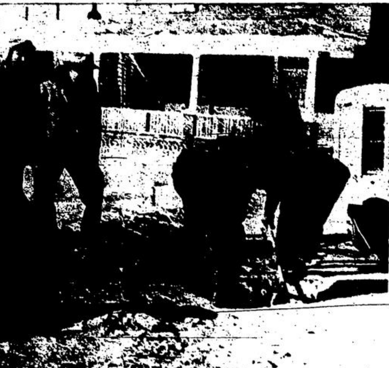
PNEUMATIC DRILLS JAB into the frozen surface of Wallace Street as efforts were intensified yesterday to locate the broken water main, eventually pinpointed near the Mill St. corner, which had cut off water to Warren Grove residents for a day and a half before the auxiliary well filled empty lines. Background centre are P.U.C. Chairman F. Oakes, and A. Duby supervising the search.
