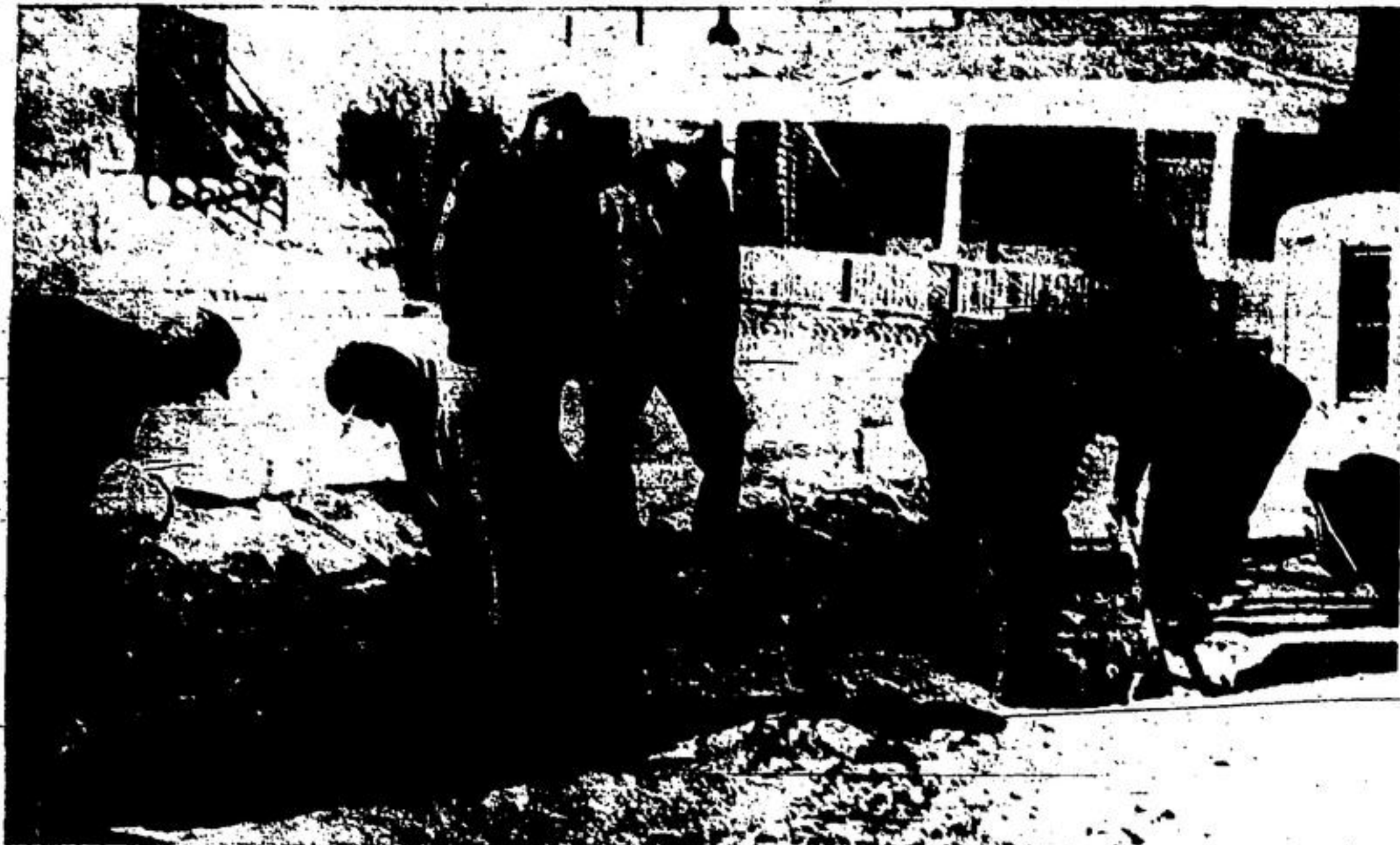
PNEUMATIC DRILLS JAB into the frozen surface of Wallace Street as efforts were intensified yesterday to locate the broken water main, eventually pinpointed near the Mill St. corner, which had cut off water to Warren Grove residents for a day and a half before the auxiliary well filled empty lines. Background centre are P.U.C. Chairman F. Oakes, and A. Duby supervising the search.
