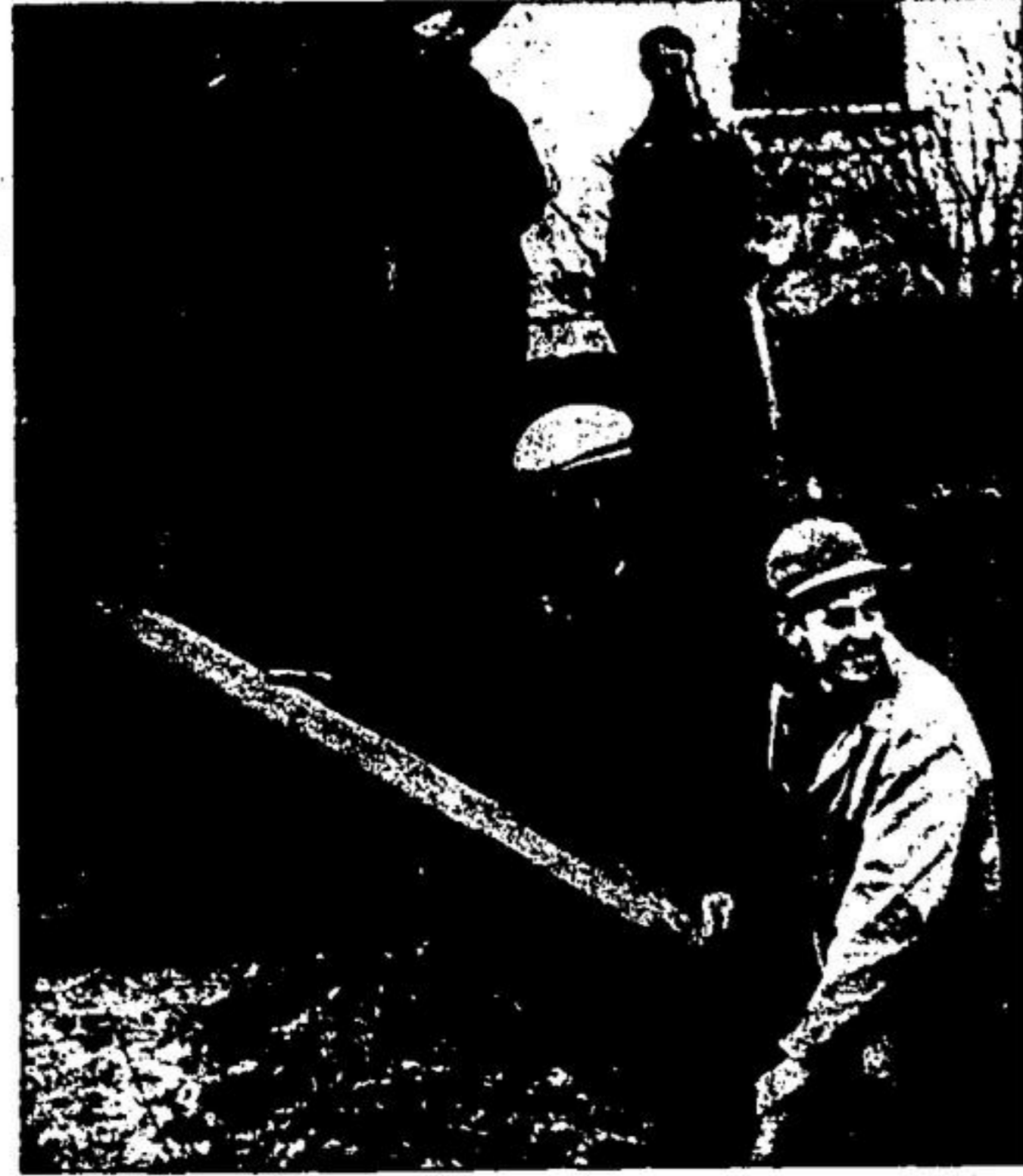
THE LAST TILE! Down it goes in Warren Grove's final sewer excavations which last week, after mud, water, bumps and general inconvenience had characterized the work since mid-summer. Here workmen pause for a smile before dropping the conduit.
