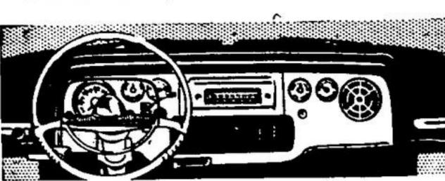
New curved instrument panel with gleaming recessed dials has the look and efficiency of an airplane flight deck! The PowerFlite automatic transmission. Flite Control lever is mounted on the dash with other controls that are seldom used.
