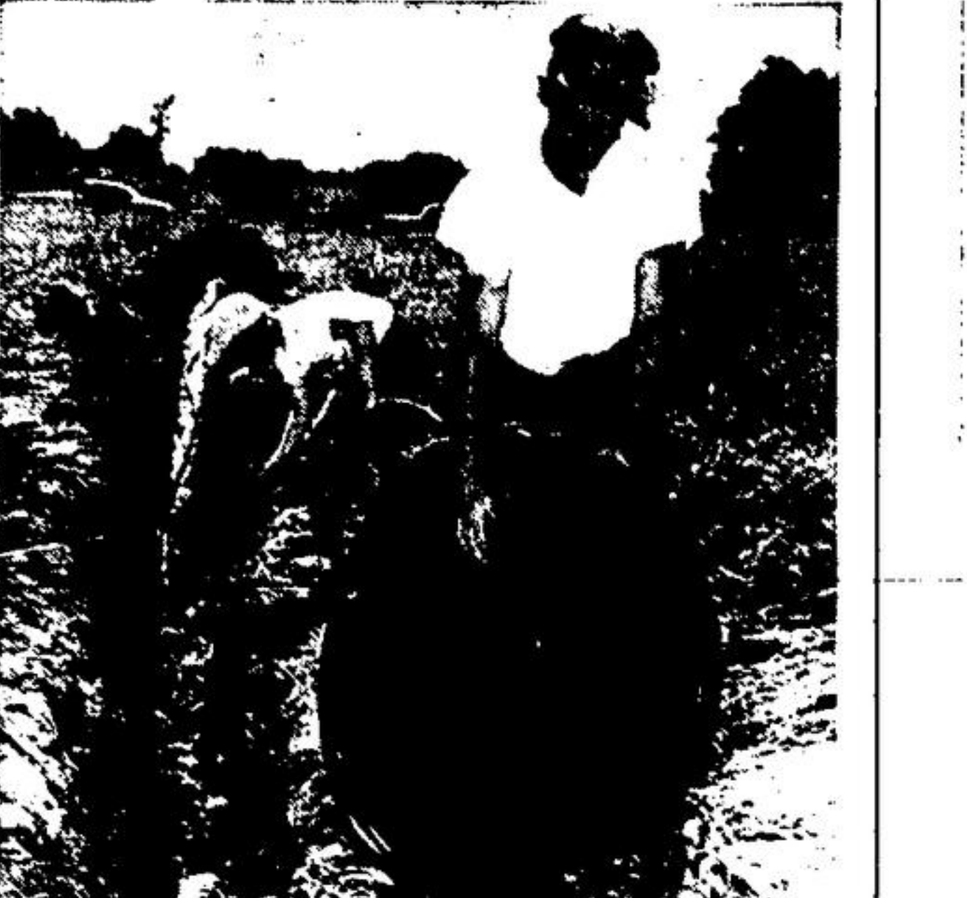
A PIPE-DREAM COMES TRUE for the man on the land. The flexible plastic C-I-L, Polythene makes pipe-laying chores a cinch. All he needs are a rough trench a saw for cutting pipe lengths and a screwdriver for tightening fittings. Flexible polythene bends around rocks, curves and corners.
