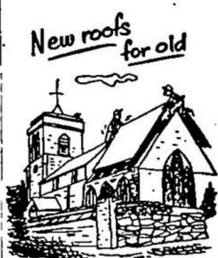
A NUMBER of ancient English churches are replacing their equally ancient roofs with aluminum. One of these is the Chapel of St. James in the village of Nether Warton, Oxfordshire. Its lead roof, originally laid in 1665, brought £478 as scrap - enough to pay the whole cost of installing the new roof.
