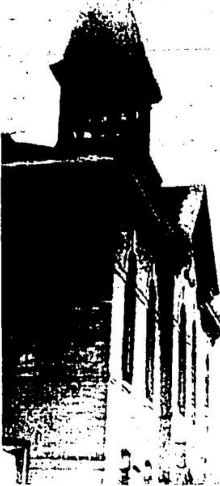
BEFORE AND AFTER scenes show Acton's decapitated tower as the town hall tower loses its steeple. Ajax workmen took the top off on Monday as the town council became wary of its weakened condition. The smaller picture shows the tower minus only some of the very point of the steeple and the larger picture shows the complete decapitation. The tower, when repaired, will remain intact to house the town bell and fire siren. The steeple will not be returned. —Staff Photo
