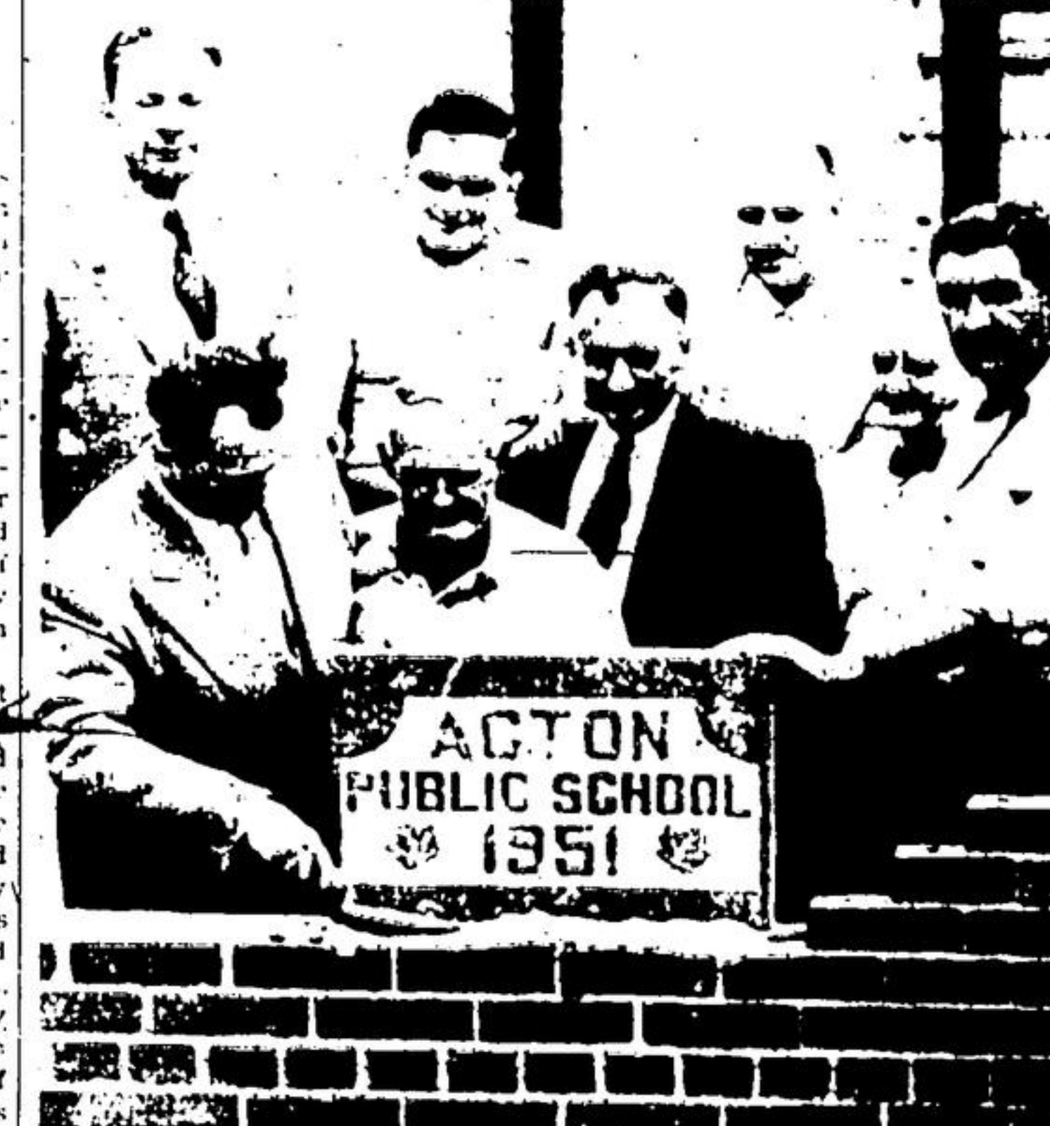
MAYOR TYLER HOISTED the corner stone into place and Chairman Oakes spread the mortar as school board officials watched the corner stone laying on the site of the $227,000 addition to Acton Public School. Shown in front are Dr. Oakes, Louis Thompson, brick layer, C. Heard. In the back are W. Wolfe, T. Watson, J. Creighton, School Board secretary-treasurer W. Middleton and Mayor Tyler. —Staff Photo
