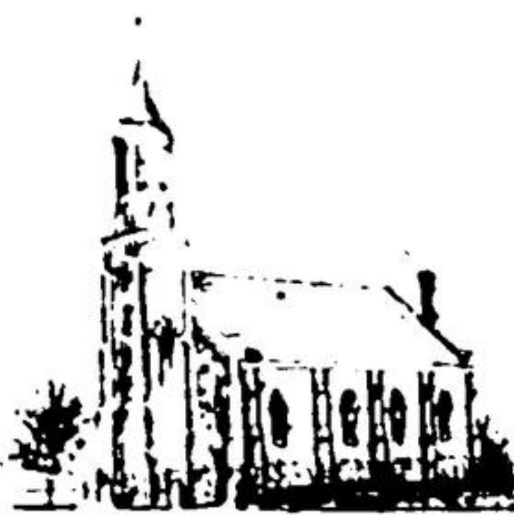
ST. JOSEPH'S CHURCH is shown prior to the removing of the steeple.
