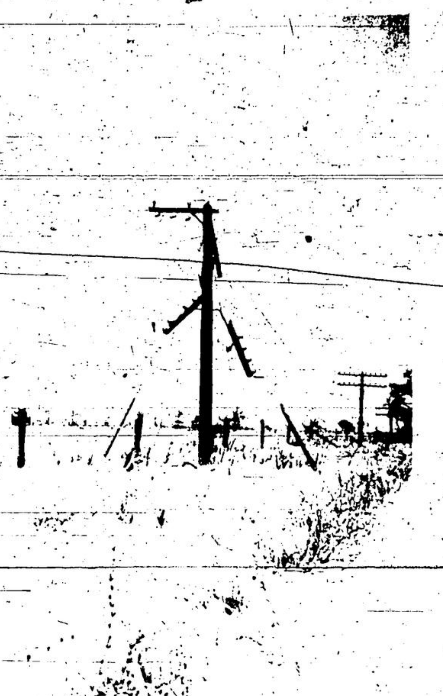
Never for years has winter's icy blast covered all with a blanket of ice, transforming the land into picturesque beauty. Although the beauty added to the hazards of motorists, it also wrecked and caused untold damage to our lines of communication. The photo above, taken on a side road in central Halton, shows a telephone pole with cross-arms fractured and wires entangled from the weight of ice. In other sections, as many as a dozen poles were flattened and workmen are laboriously toiling to resume service.
