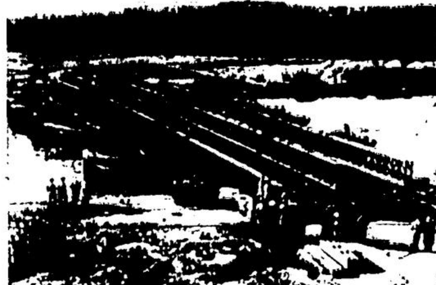
The Bailey bridge is the best answer yet to the enemy's demolitions, and greatly facilitated Allied advances in both Italy and Normandy. It is a British invention and is named after its inventor, Mr. D. C. Bailey of the Ministry of Supply. Components, which are made both in the U.S.A. and Britain, are interchangeable and can be speedily put together. This together with its great strength and stability make it ideal for every purpose for which heavy bridging is required. Picture shows a Bailey bridge built across a river somewhere in Britain.
