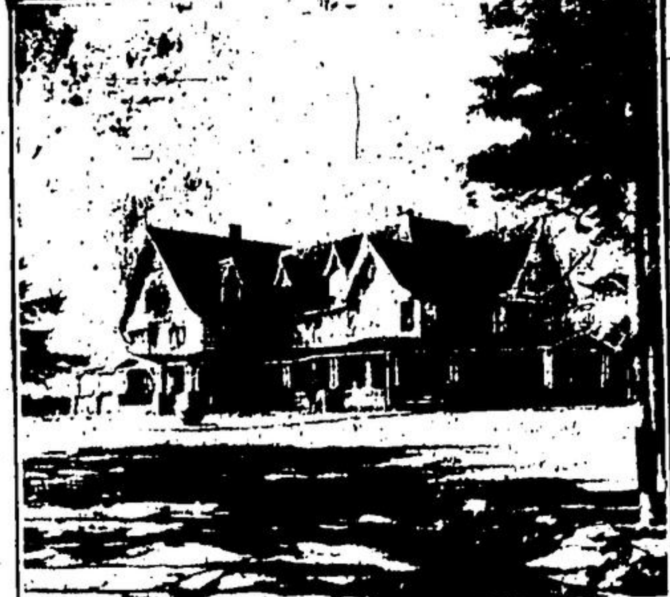
Dulany House and Grounds (Administrative Buildings) Prince Edward Island National Park, Prince Edward Island, Canada.
