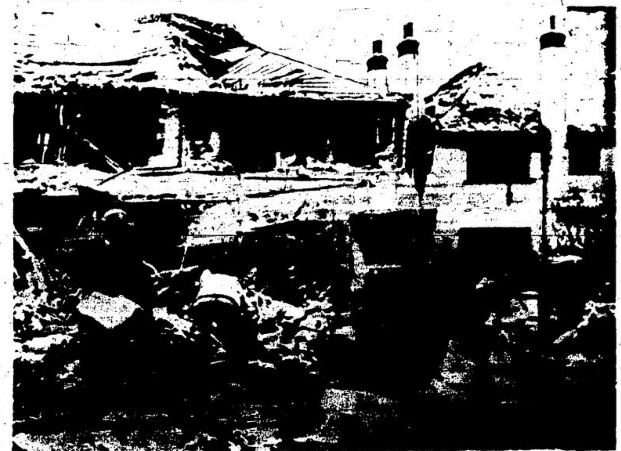
These wrecked houses are some of the 50 destroyed by the explosion and fire when a German Heinkel bomber, loaded with bombs, fell at Clacton, on the Essex coast. The mines were detonated by the impact of the crash. Three civilians were killed and more than 100 injured. The bombing plane was blown to bits and the four German fliers died.
